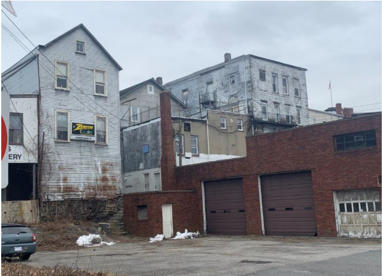
Buildings in disrepair on Bank Street
