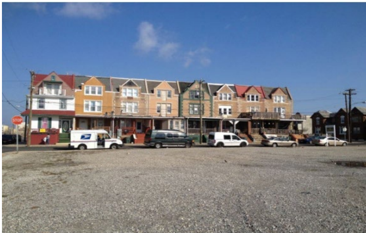
Housing in the Inlet Neighborhood to be rehabilitated with NRTC funds
