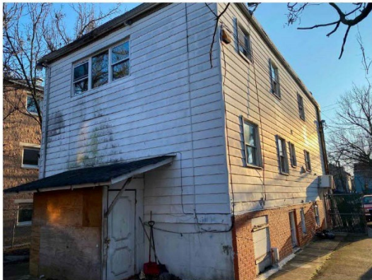
Picture 2: Current building at 293 Townsend St property. Will be demolished and replaced with 6-unit new building (Objective 3).
