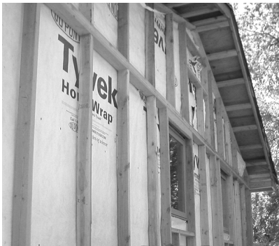
Frame wall for insulation: Technicians fastened a frame wall with brackets that place the wall away from the existing exterior wall by a half inch so that the sprayed foam can flow behind the studs and plates to reduce thermal bridging.
