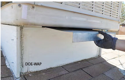
Winter slide damper: May exist somewhere in the cooler. Insert for winter season. Remove for summer.
