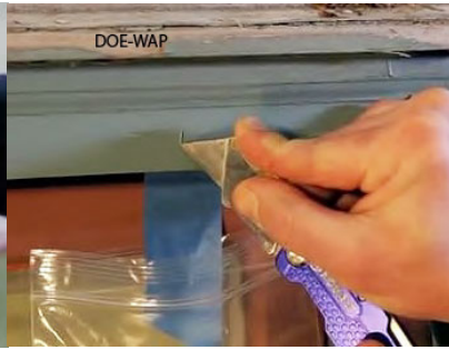
Cut through all the layers of paint. Also install a bag beneath the cut to catch paint fragments.
