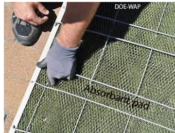
Cooler pads: Pads collect dirt and scale. Replace them when cleaning is ineffective.
