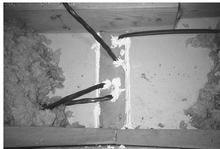
Leaky top plates: The cracks along top plates are from lumber shrinkage. They are small cracks but there are long lengths of them.
