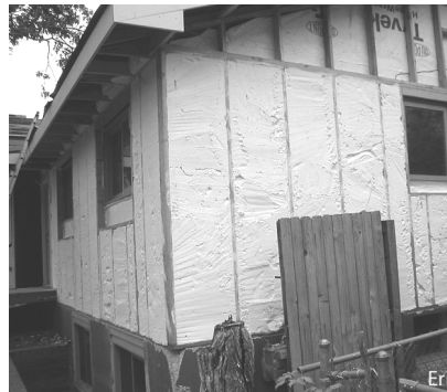
Open-cell polyurethane foam: The foam was sprayed into the cavities and the excess shaved off. New sheathing, house wrap, siding, and windows follow later.
