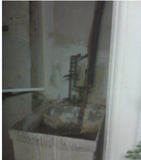
Work Sink with A/C Discharge
