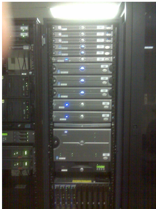
Data Center Servers
