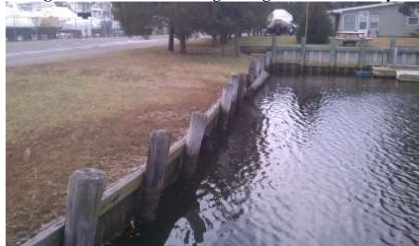
Figure 12: Bulkhead Damage along South Boom Way
