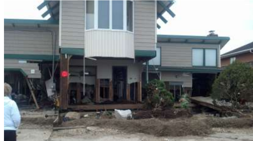
Figure 4: Damaged Residential Structure
