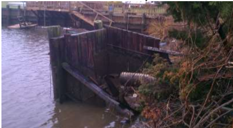
Figure 10: Bulkhead and Drainage Damages along West Calabreeze Way
