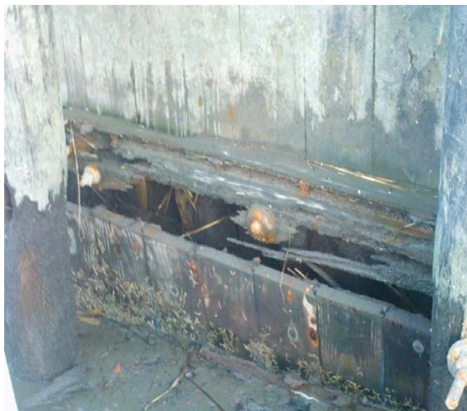
Figure 25: Amherst Avenue Bulkhead Decay
