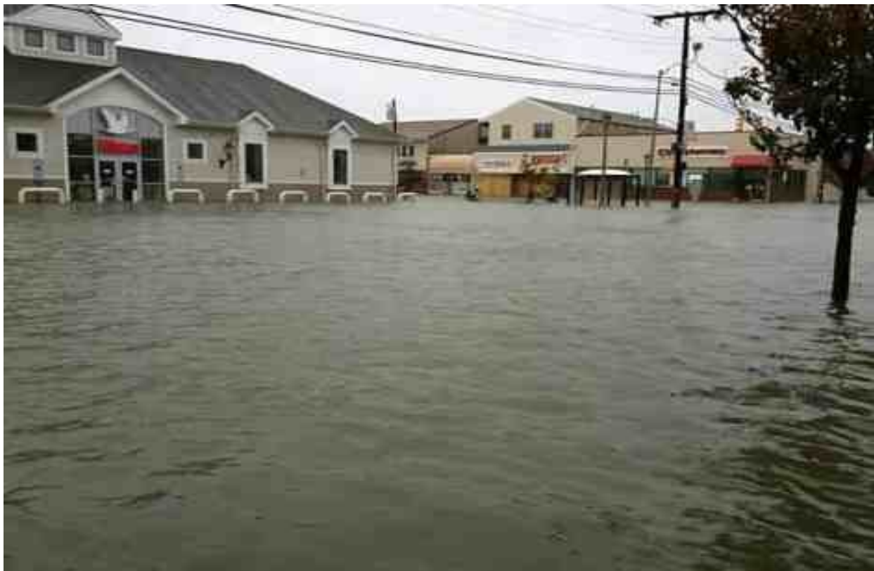
Figure 5: Superstorm Sandy Damage in Downtown Margate at the Intersection of Washington Avenue and Ventnor Avenue
