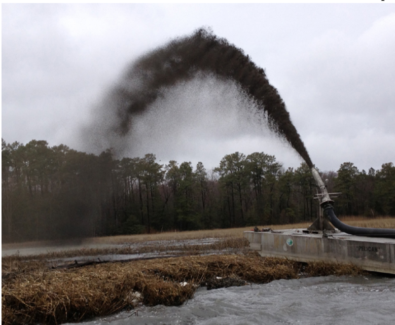
Figure 26: Thin Film Spraying of Wetlands Areas
