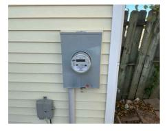
Service Amperage: Service Amperage 150amps 120/240VAC Service Amperage: Service Entrance Conductors Type 2/0 Aluminum
