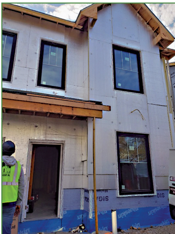
Madison Family Apartments – Madison, New Jersey Insulated Envelope and Low Solar Heat Gain Value Windows
