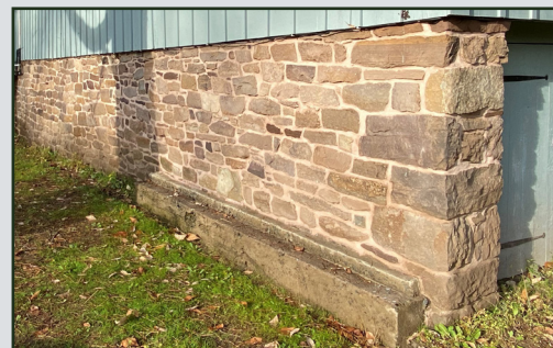
Restoration of stone foundation.
