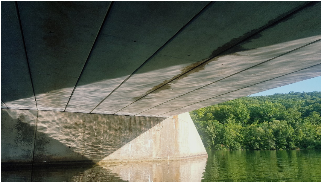
Figure 1. Bridge over the Monksville Reservoir, where more than 100 Myotis bats were found roosting in the expansion joints. Note the obvious urine marks along the most occupied joint.
