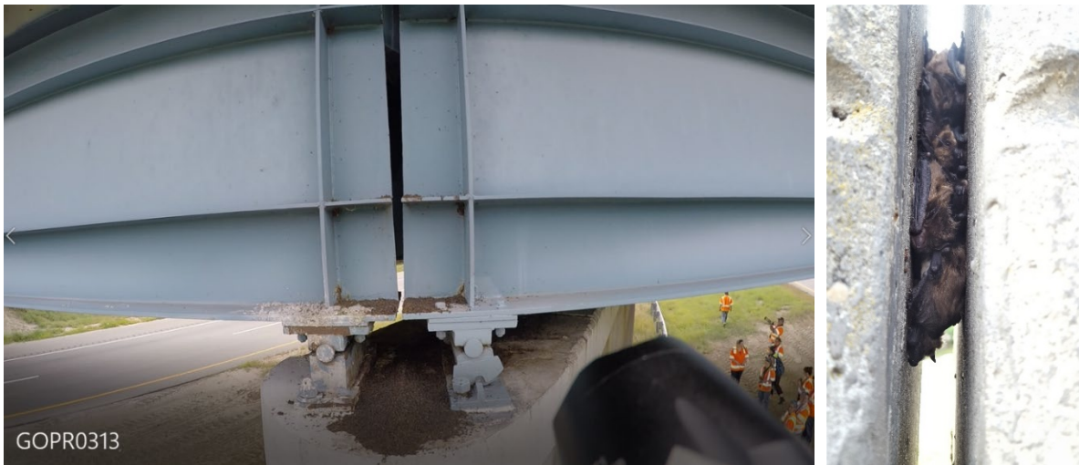
Figure 1. Bridge inspection field training with the US Fish and Wildlife Service and NJ Department of Transportation. At left, a remote-controlled camera on a telescoping pole captures images of bat guano on the pier cap; at right, big brown bats roosting in a parapet gap of the same bridge in Millville, NJ.
