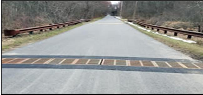
*The surface of a roadway on the Assunpink WMA in Upper Freehold Township. Underneath the grating are tunnels to prevent wildlife from crossing the asphalt.*
