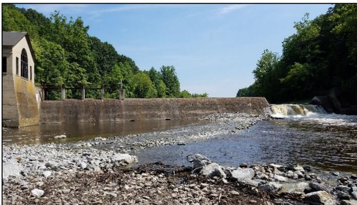
*The 18-foot high, 330-foot long dam constructed in 1909 had become an impediment to migrating fish.*
