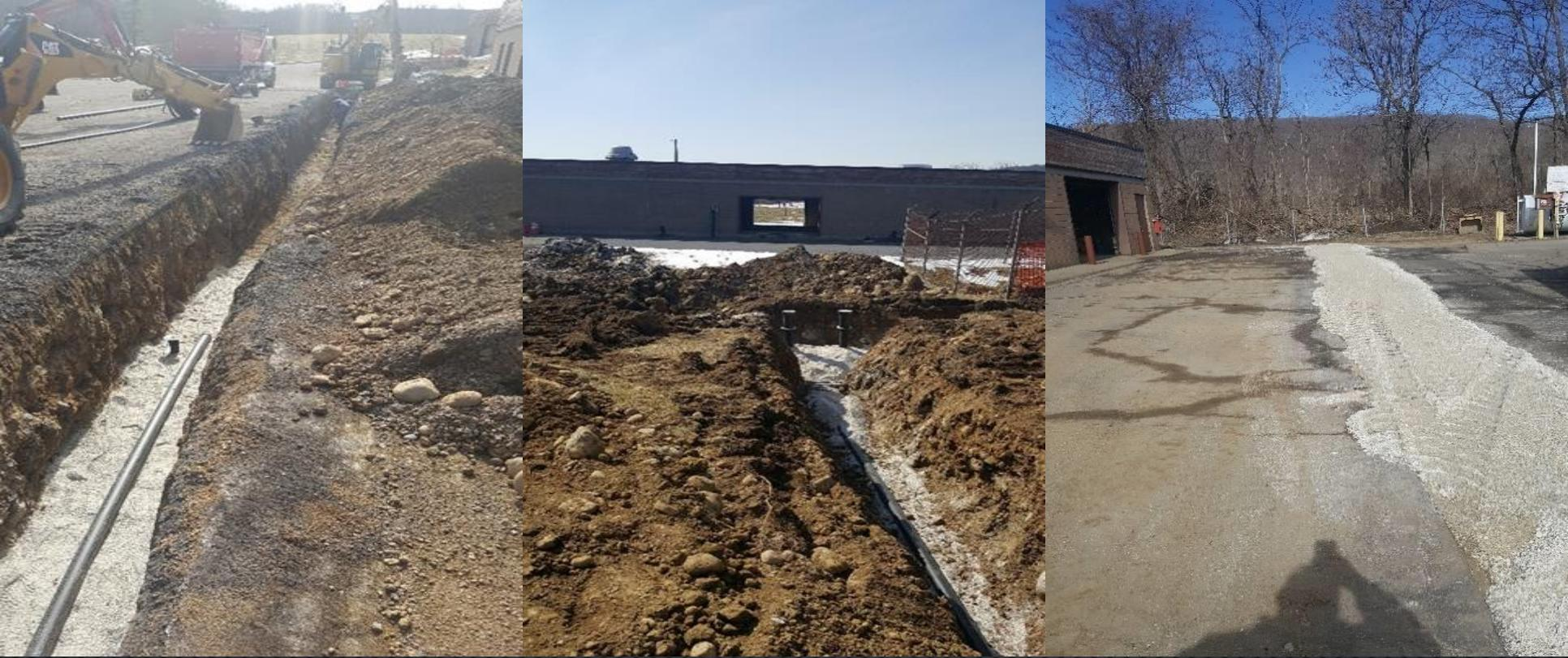
The Domestic Waterline Project started as soon as the snow was off the ground in the Spring of 2021. This project replaced the old brittle PVC-line that had several failures in recent years. The domestic waterline was replaced throughout the entire Pequest facility. This project was covered by Corporate Business Tax (CBT) funding costing \$422,869.90
