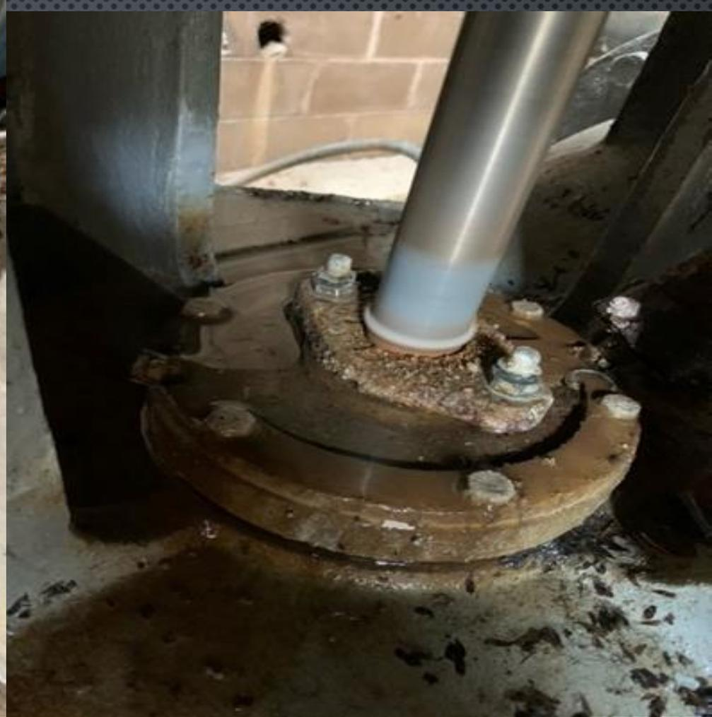
Wells #1 and #5 were also serviced because the packing was leaking around the shafts and there was no more adjustment left. New packing glands were installed which is labor intensive because the motors need to be pulled by a hoist truck. The cost was about \$8,000 dollars.
