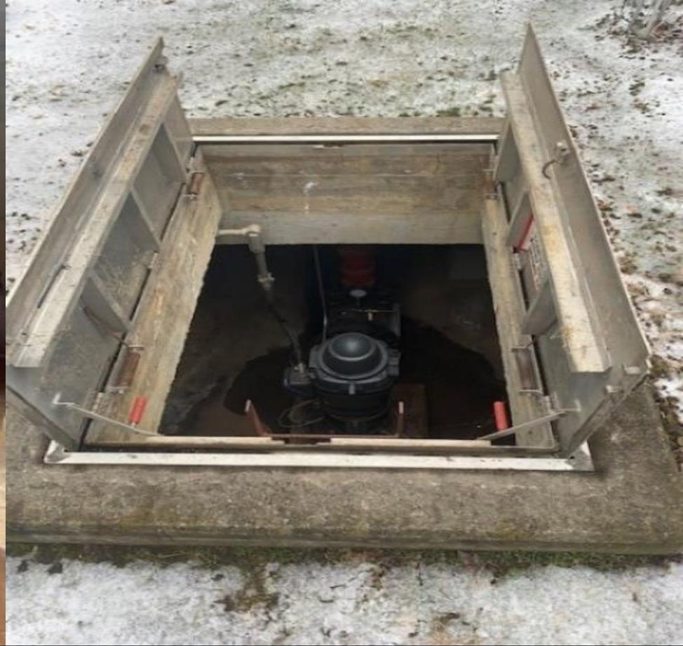
Well #3 was rebuilt during 2021 because do to a 200 gallon per minute pumping decrease which is usually a sign of impending failure. This well is needed along with several other wells to maintain trout production year-round at the facility. When it was taken apart the impeller was almost worn to nothing. Several components are replaced during a rebuild and the project cost \$29,450 covered under CBT funding.
