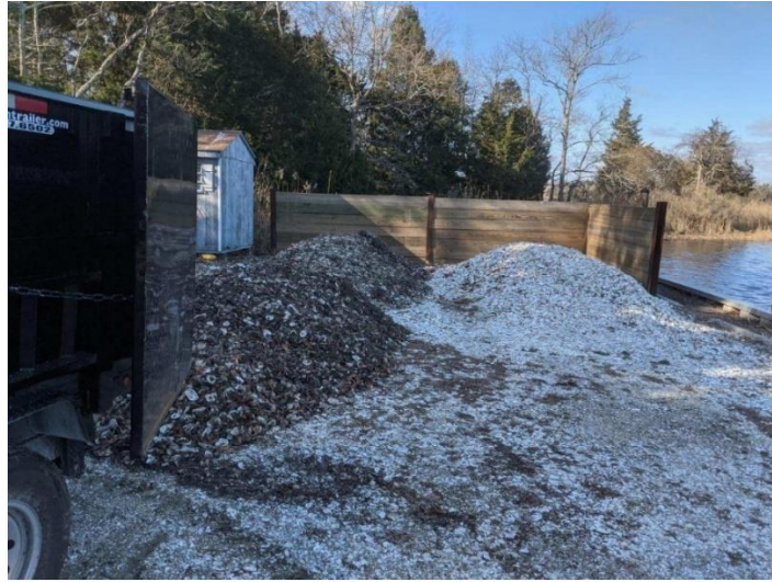
Short term storage/staging area
