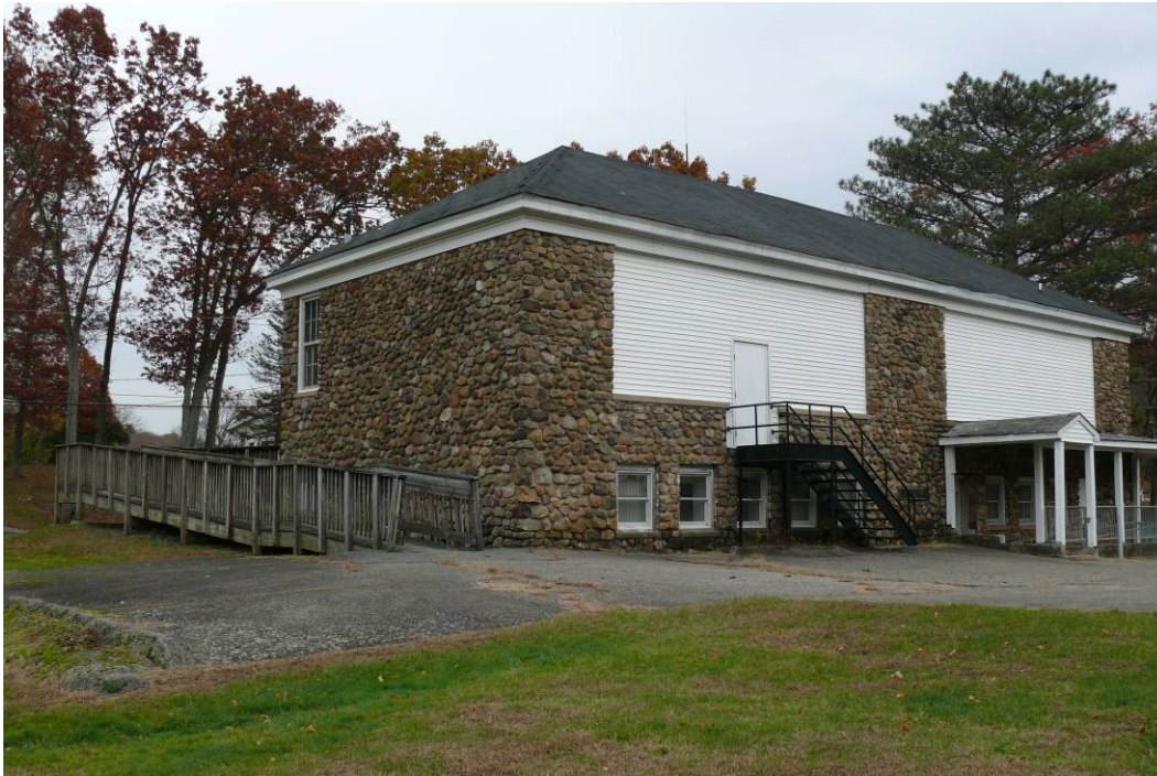
Photo 0005: Overall view of the west and south elevations; camera facing northeast.
