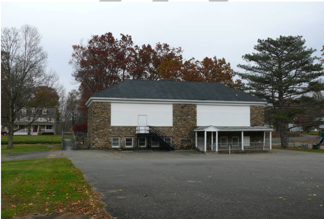
Photo 0006: Overall view of the rear (south) elevation; camera facing north.
