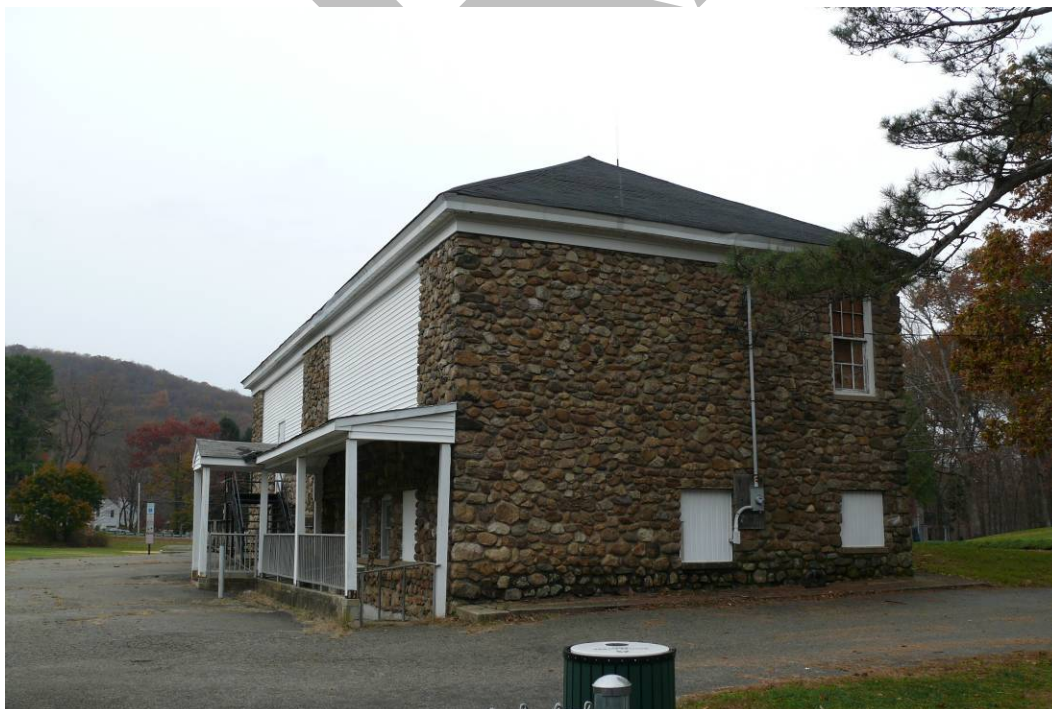
Photo 0004: Overall view of the east side elevation; camera facing northwest.
