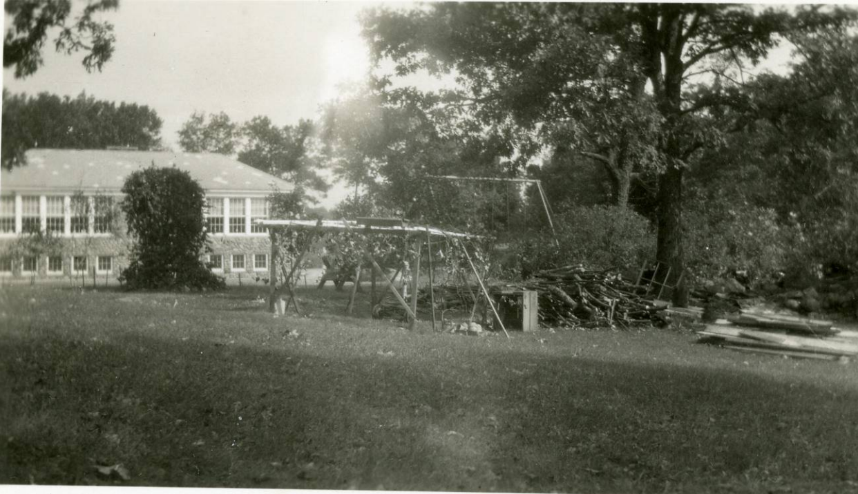
Figure 3. Early-to-mid-twentieth-century view showing the rear of Lafayette School. Note the second-floor bands of windows that are currently obscured by vinyl siding and the basement level before the current entrance was added. 3
