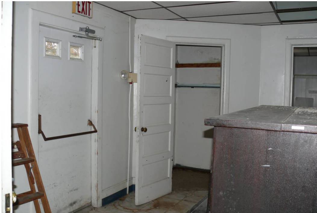
Photo 0009: Overall view of the entry vestibule; camera facing east.
