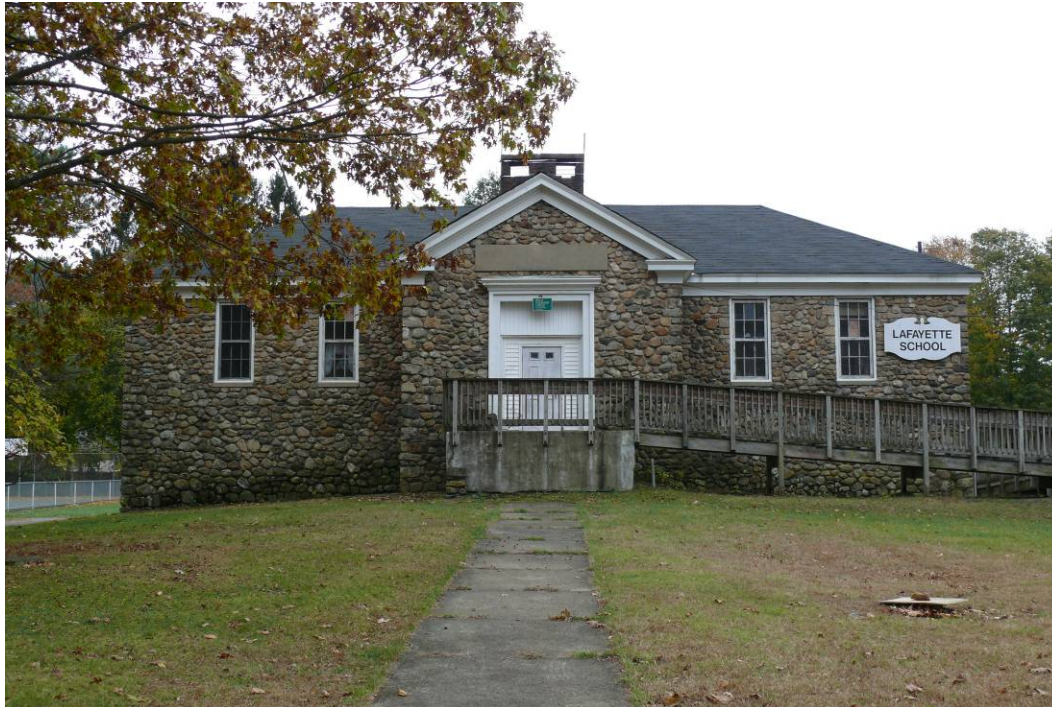
Photo 0001: Overall view of the front (north) elevation of Lafayette School; camera facing south.
