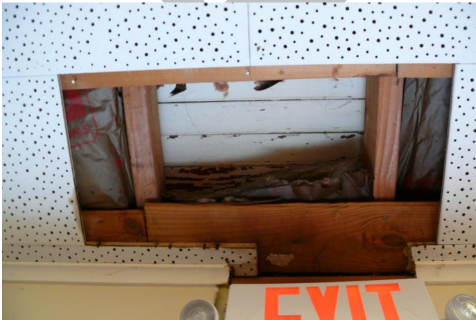
Photo 0018: View showing early beaded board ceiling intact above mid-twentieth-century finishes at the second floor; camera facing up.
