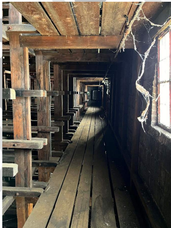
Photo 50. Interior view of Bonded Warehouse 1B barrel ageing rack room in the 1934 section of the building (Volume A). Camera facing south (November 17, 2023).
