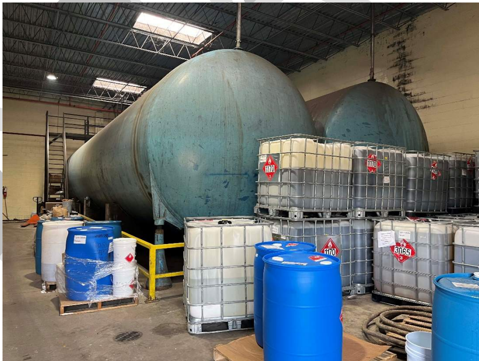
Photo 62. Interior view of the Current Bottling Plant, large storage tanks, camera facing southwest (November 17, 2023).
