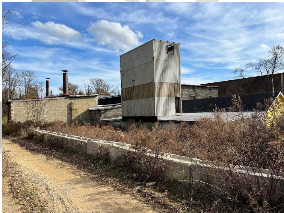
Photo 32. Exterior view of the Still House (right) and attached distillery equipment rooms (left), camera facing southeast (November 17, 2023).
