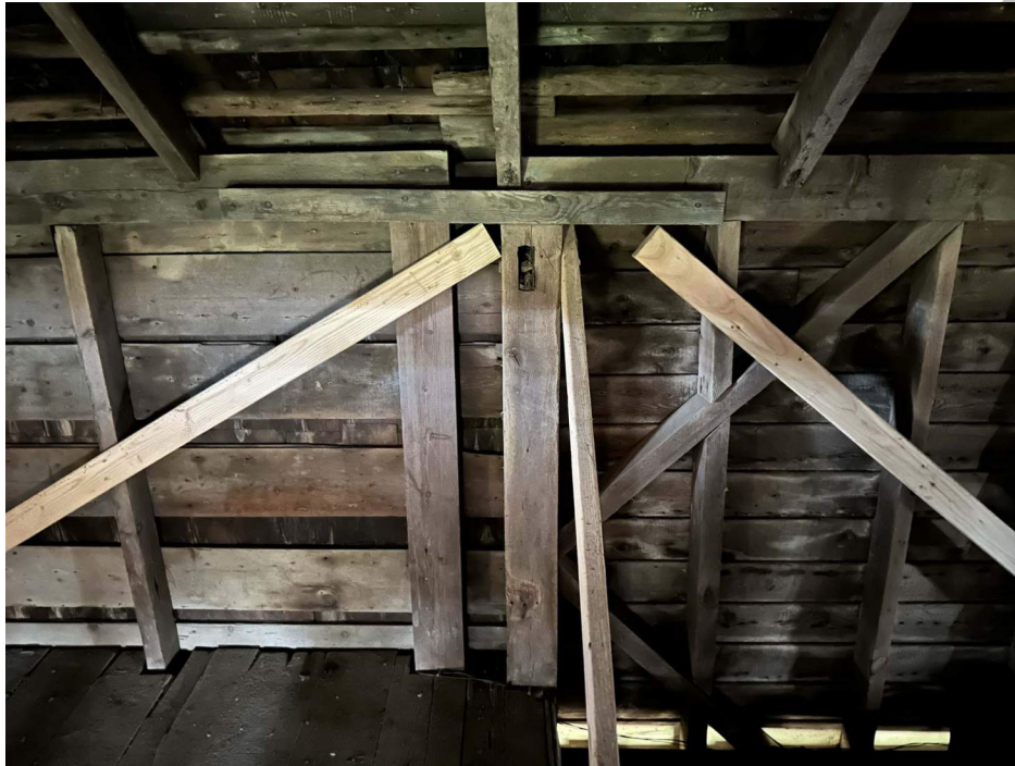
Photo 23. Interior view of the Barn, second floor structural transition from Volume A (left) to Volume B (right) of the Barn, camera facing west (November 17, 2023).
