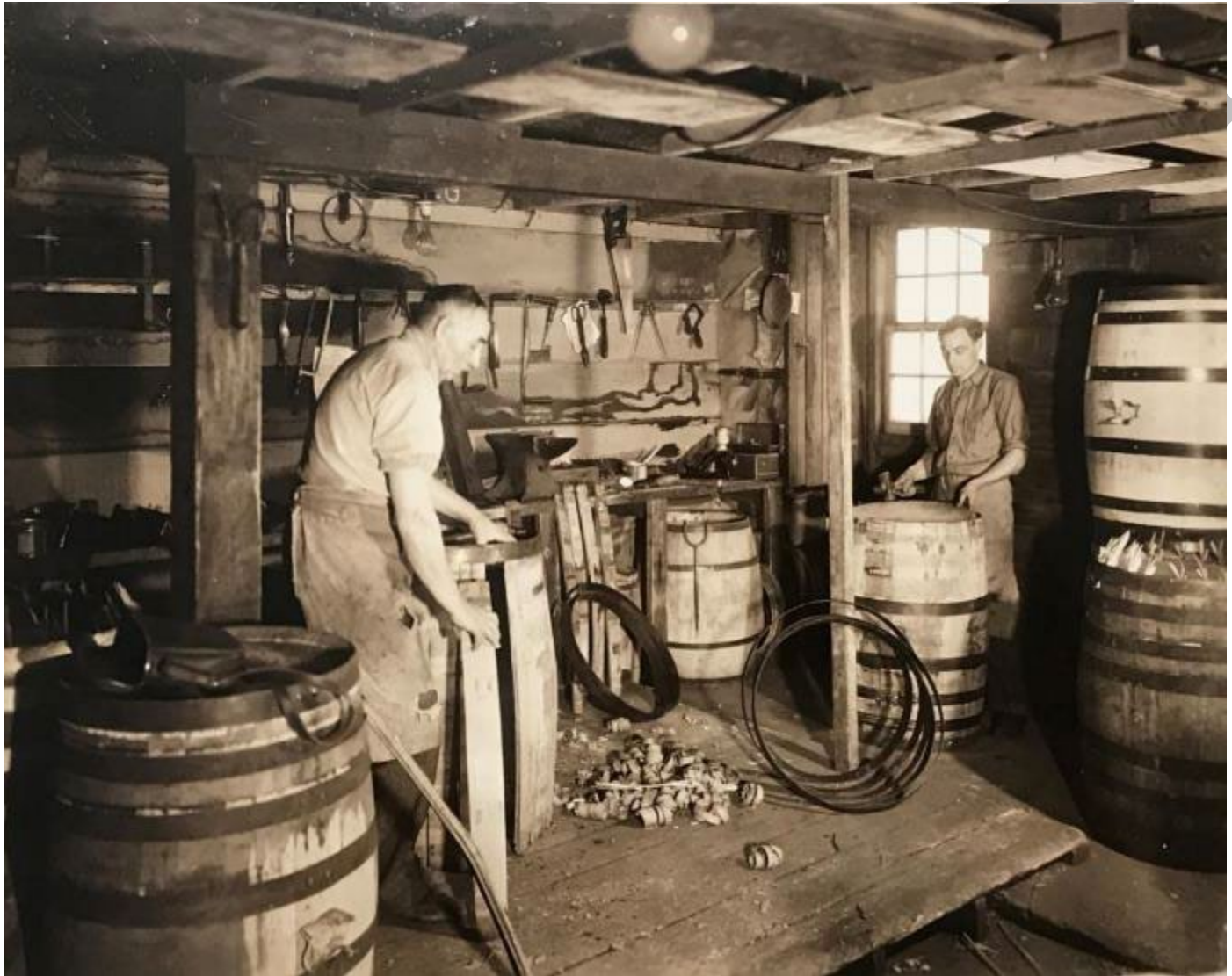
Figure 19. Barrel construction in the Cooperage Shop, which was located in the existing Barn, 1930s. (Source: Laird & Company Archive.)
