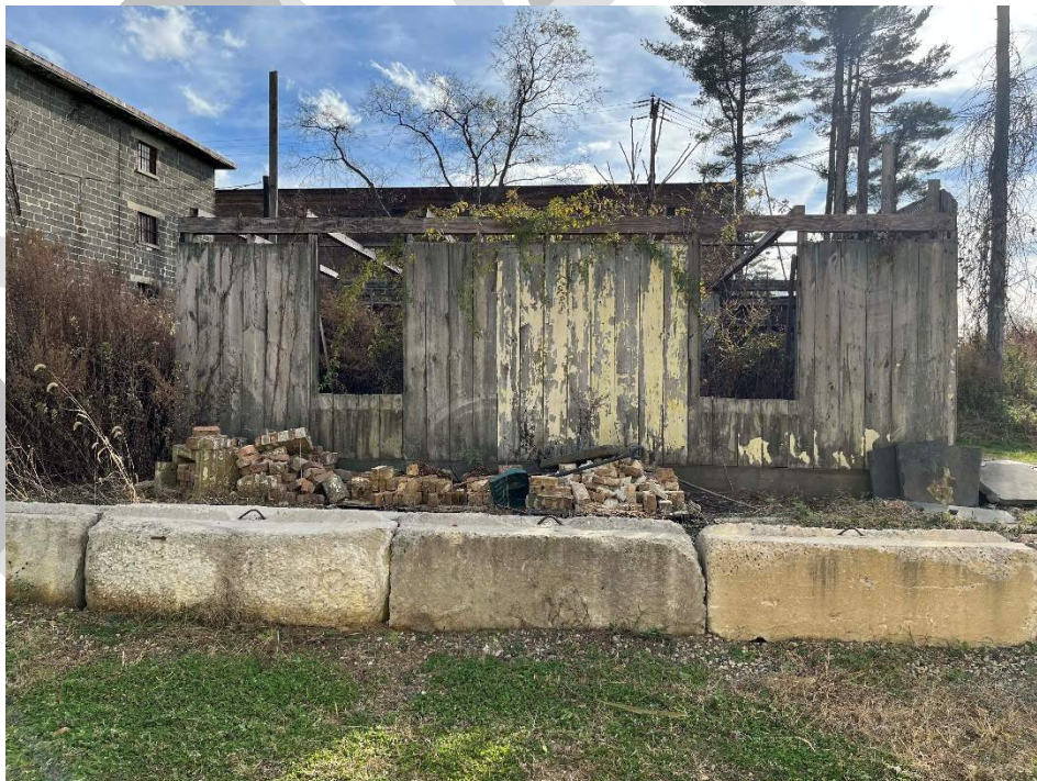
Photo 28. Exterior view of the Office, north elevation, camera facing south (November 17, 2023).
