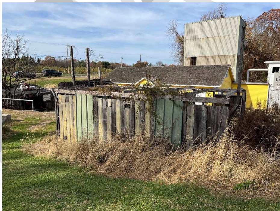
Photo 26. Exterior view of the Office, south elevation, within the surrounding context of the distillery complex, camera facing northwest (November 17, 2023).
