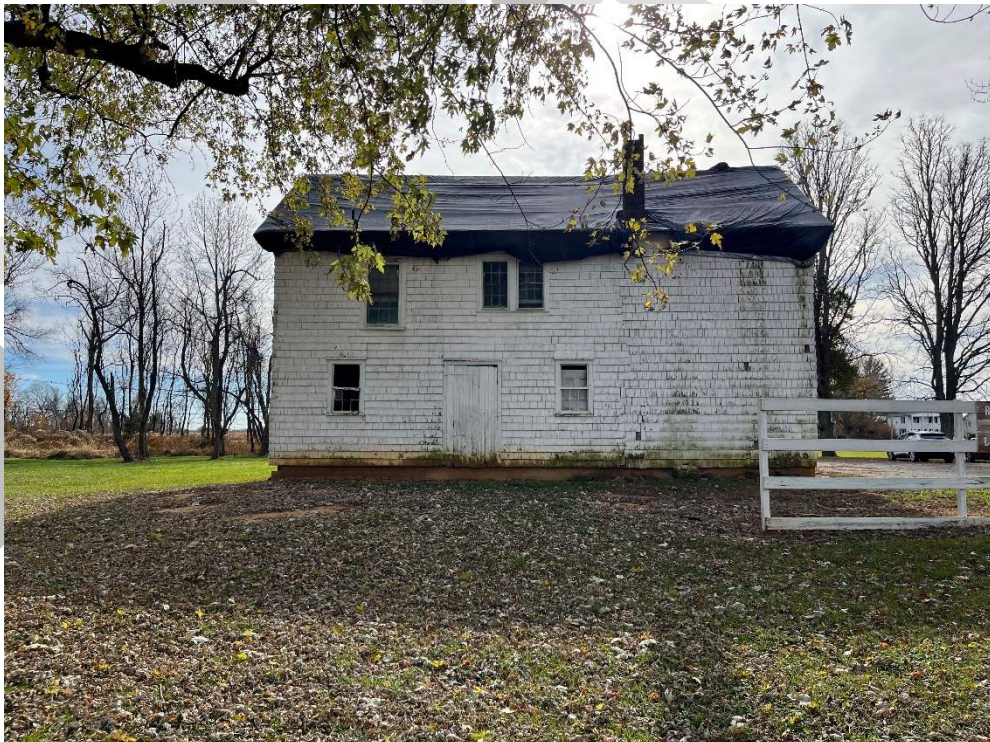
Photo 16. Exterior view of the Barn, north elevation, camera facing south (November 17, 2023).
