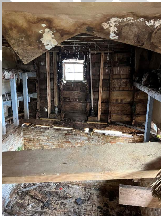
Photo 18. Interior view of the Barn, southernmost room of the first floor in Volume A above the brick root cellar, camera facing east (November 17, 2023).
