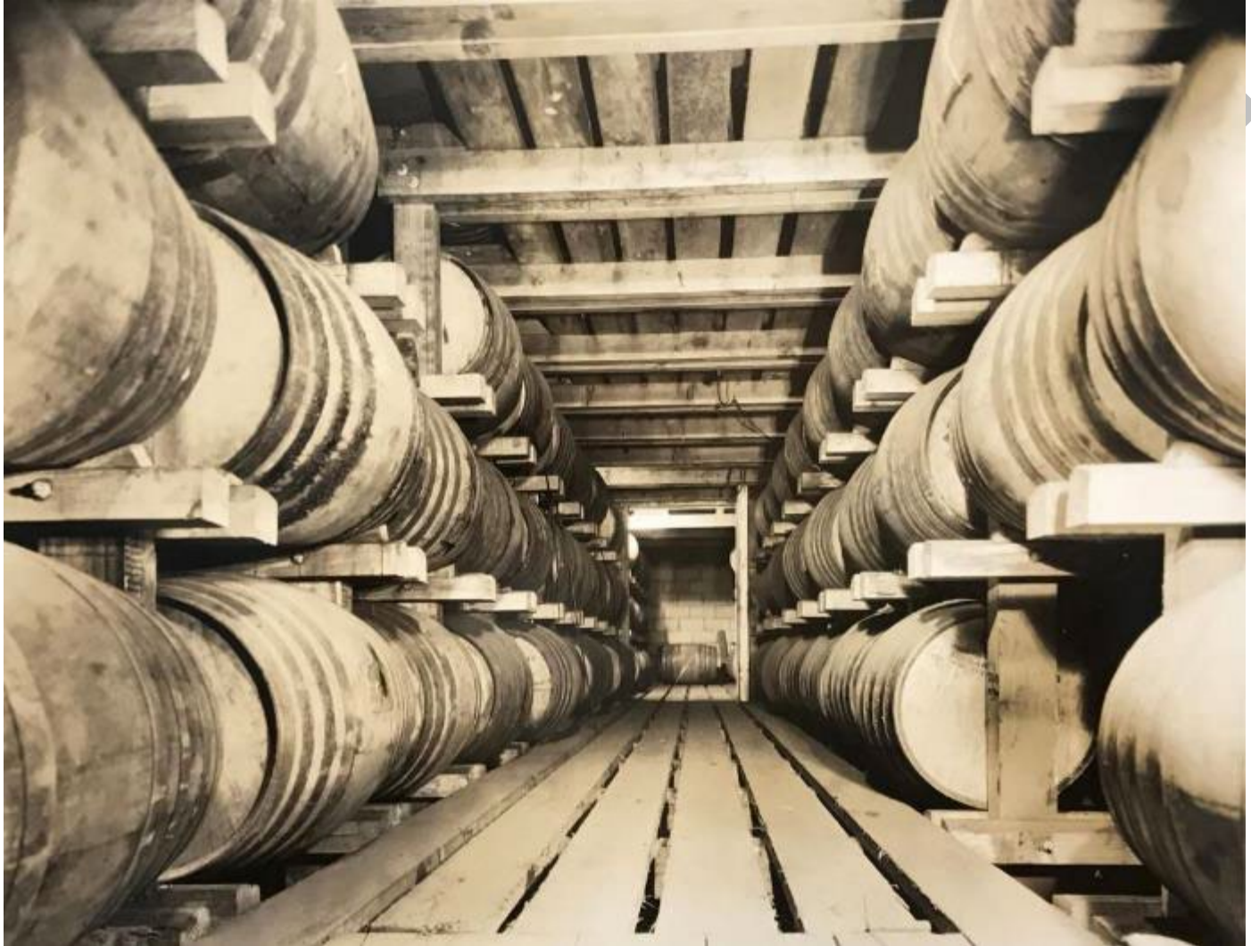
Figure 16. Interior of one of the Bonded Warehouses with barrel ageing racks, 1934. (Source: Laird & Company Archive.)
