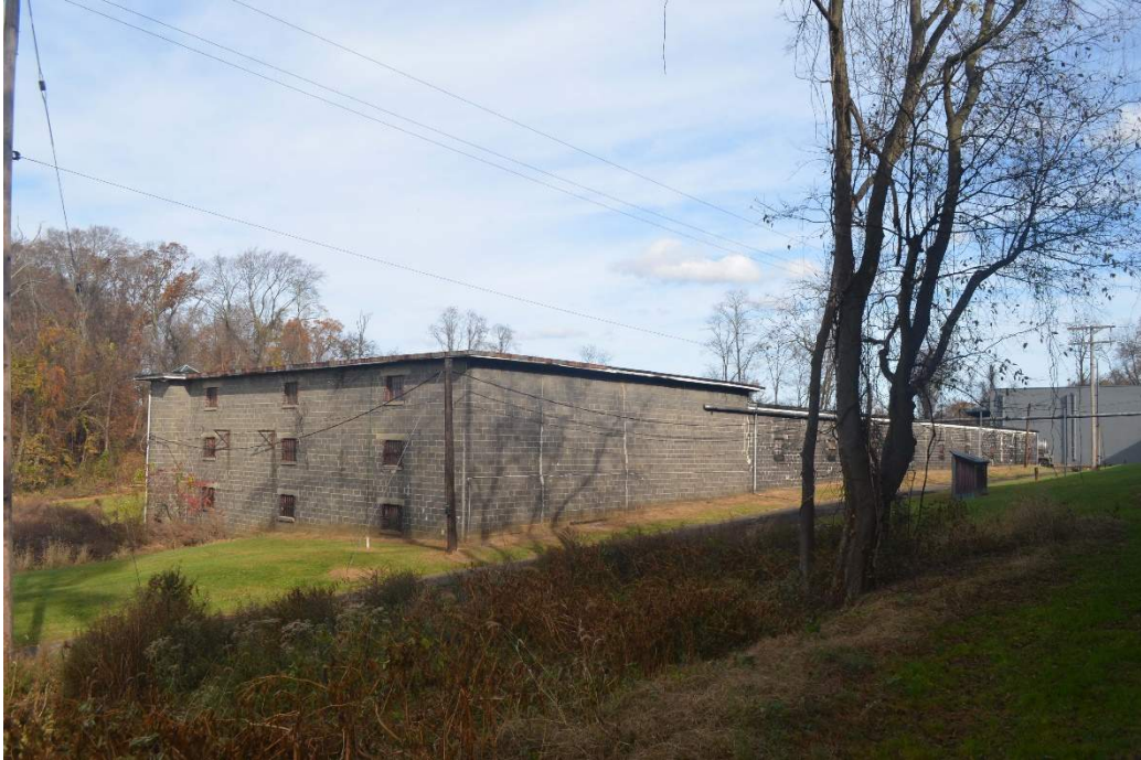
Photo 47. Exterior view of Bonded Warehouse 1B, south and west elevations, camera facing northeast (November 17, 2023).
