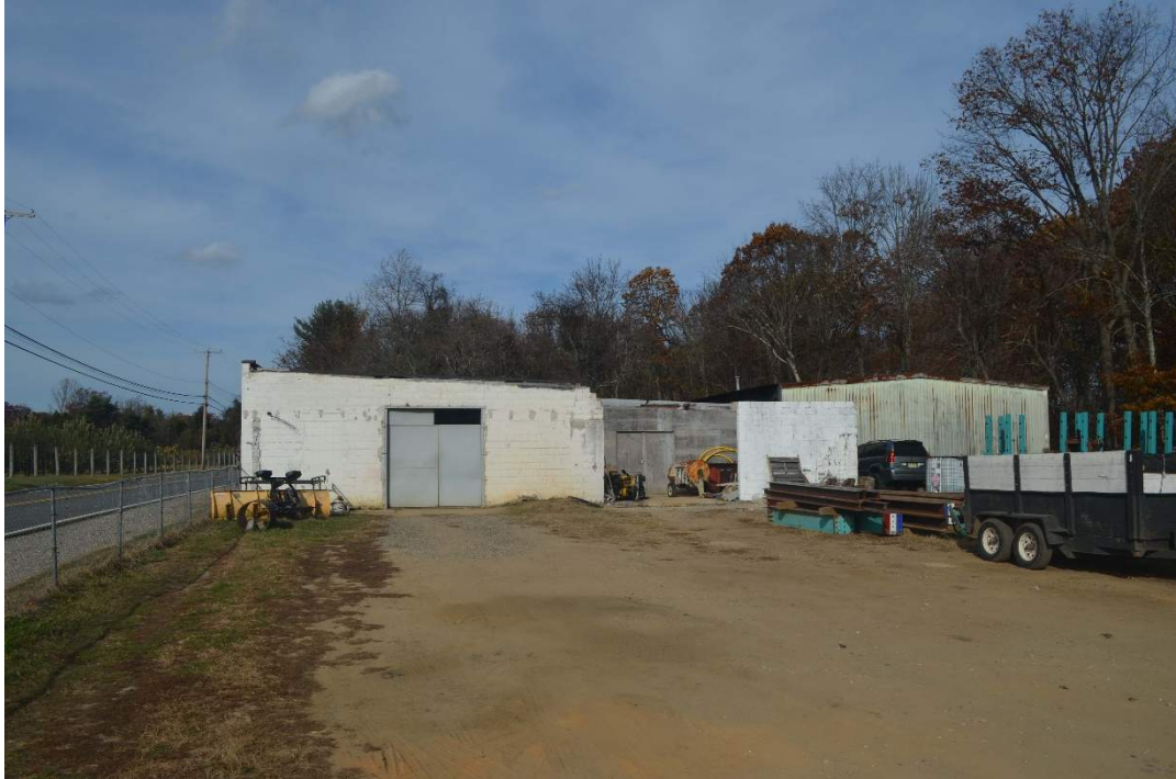
Photo 41. Exterior view of the Former Bottling Plant, south elevation, camera facing north (November 17, 2023).
