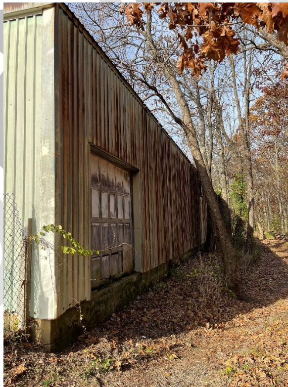
Photo 44. Exterior view of the Former Bottling Plant, east elevation of Volume B, camera facing northwest (November 17, 2023).
