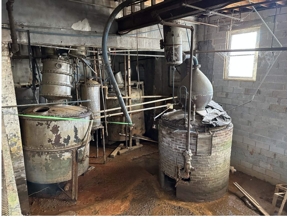
Photo 39. Detail view of historic still and kettle used for applejack distilling, with additional equipment and piping beyond, located inside the Still House, camera facing southwest (November 17, 2023).
