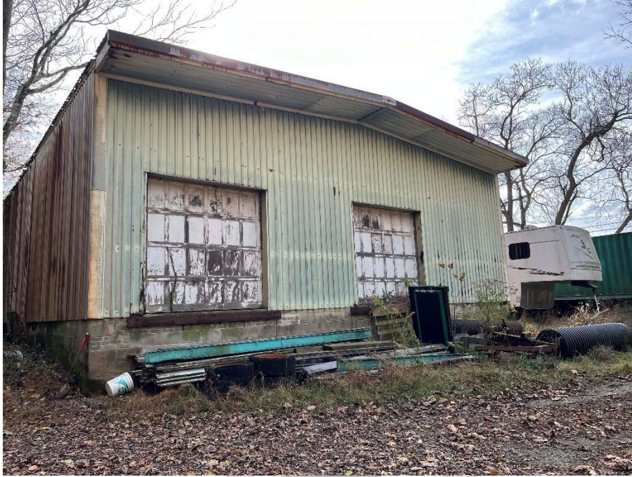
Photo 45. Exterior view of the Former Bottling Plant, north elevation of Volume B, camera facing southwest (November 17, 2023).
