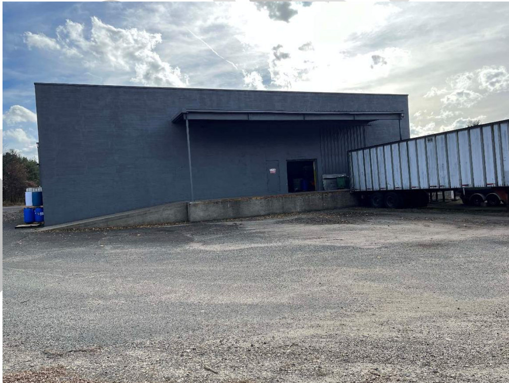
Photo 56. Exterior view of the Current Bottling Plant, north elevation of easternmost building, camera facing south (November 17, 2023).
