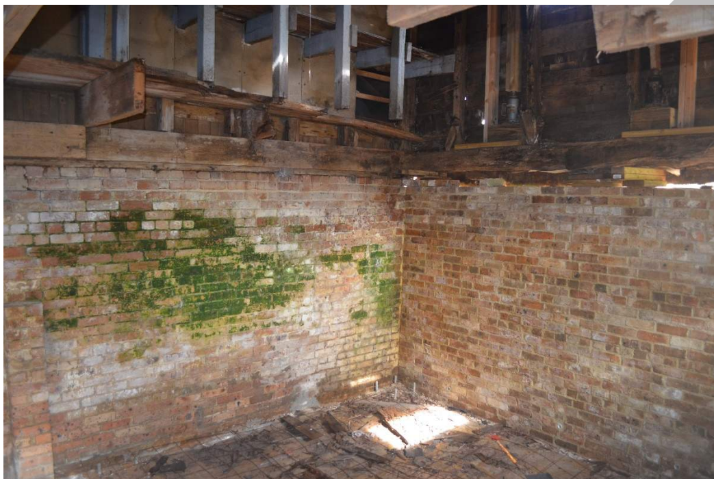
Photo 19. Interior view of the Barn, root cellar and exposed foundation walls beneath the oldest section of the Barn, camera facing northeast (November 17, 2023).
