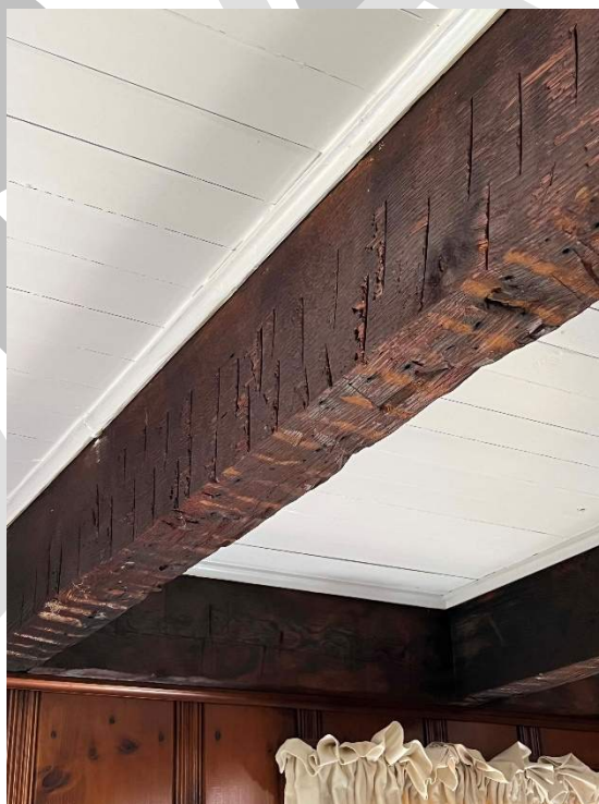
Photo 10. Detail view of the original wood beams and ceiling finish in Volume A, camera facing south (November 17, 2023).
