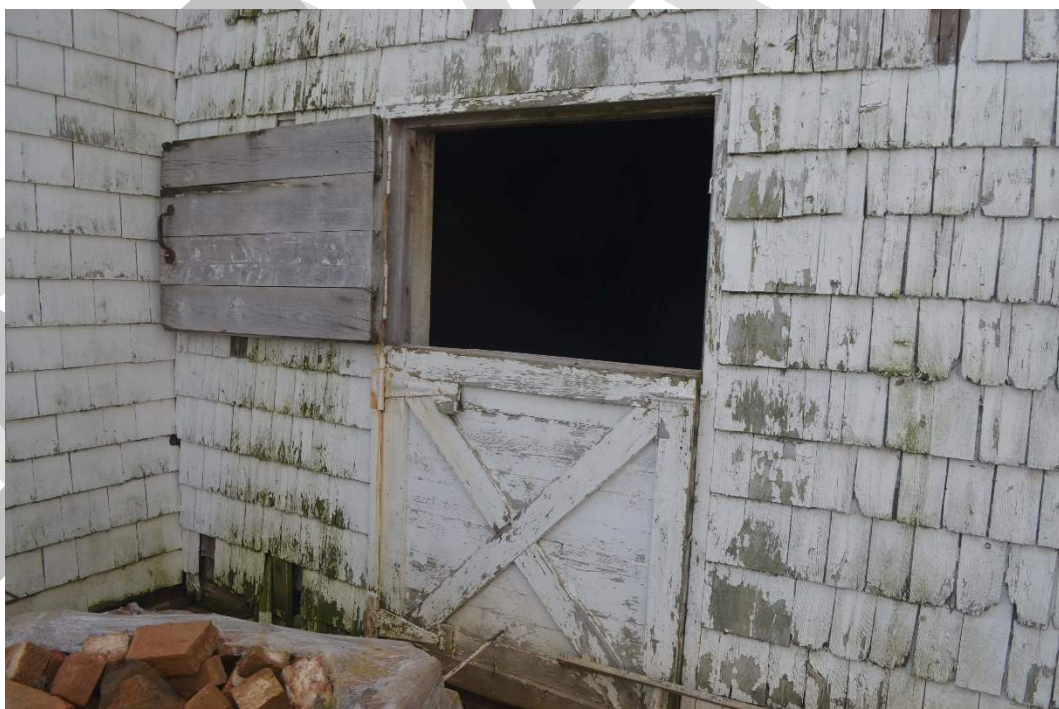
Photo 20. Exterior view of the Barn, Dutch door leading to former stable located in the middle section of the Barn (Volume B), camera facing southwest (November 17, 2023).
