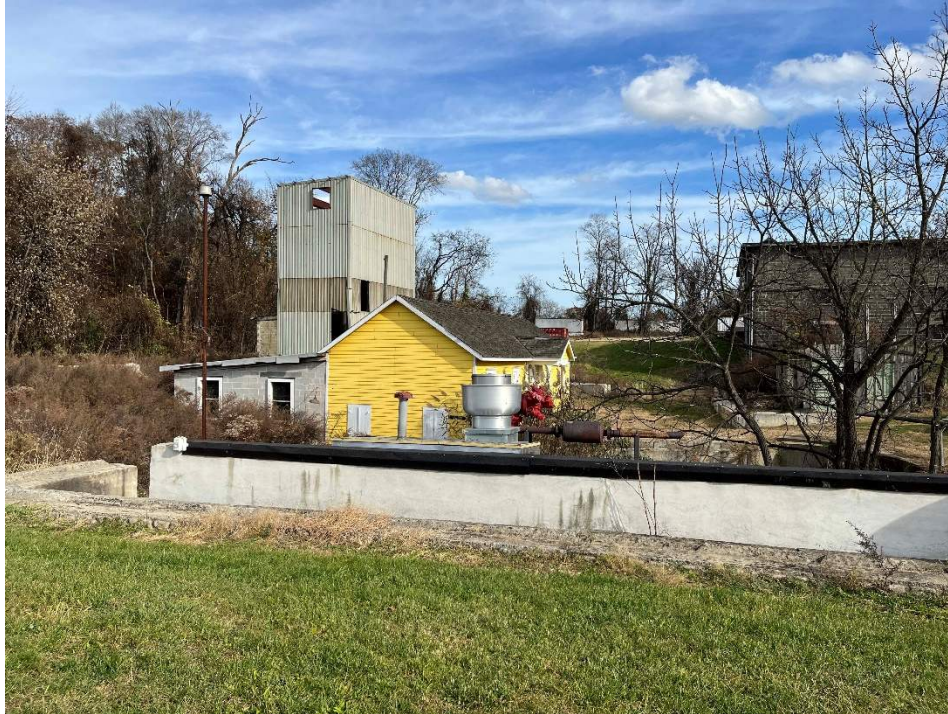
Photo 31. Exterior view of the Still House, west elevation with rear concrete block addition and attached distillery equipment buildings beyond, with Mechanical Equipment Shed in the foreground, camera facing east (November 17, 2023).
