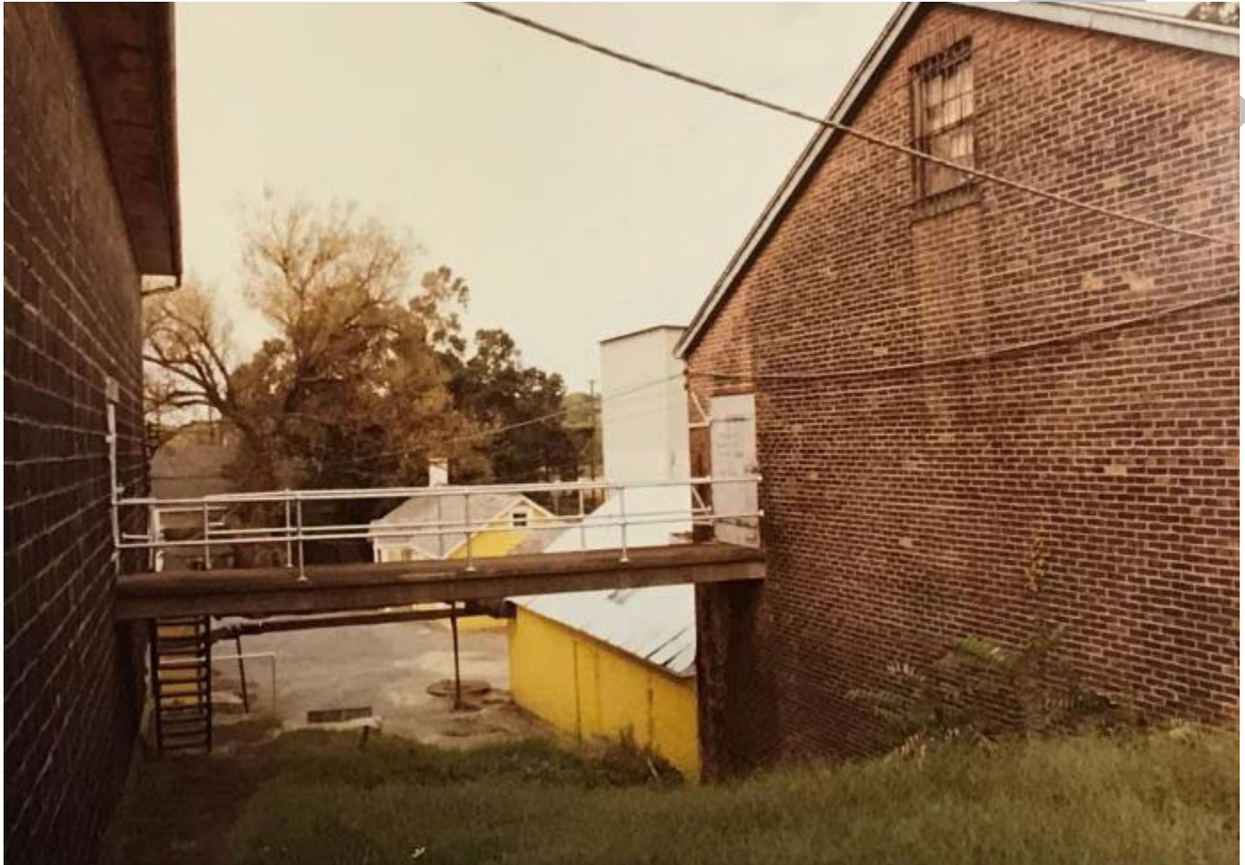
Figure 27. The 1934 Bonded Warehouse (left) and the brick Bonded Warehouse No. 1A (right, demolished) in the 1970s, looking west. The Still House is visible in the background. The steel and metal tank enclosure, which extends from the rear roof, has been constructed. (Source: Laird & Company Archive.)
