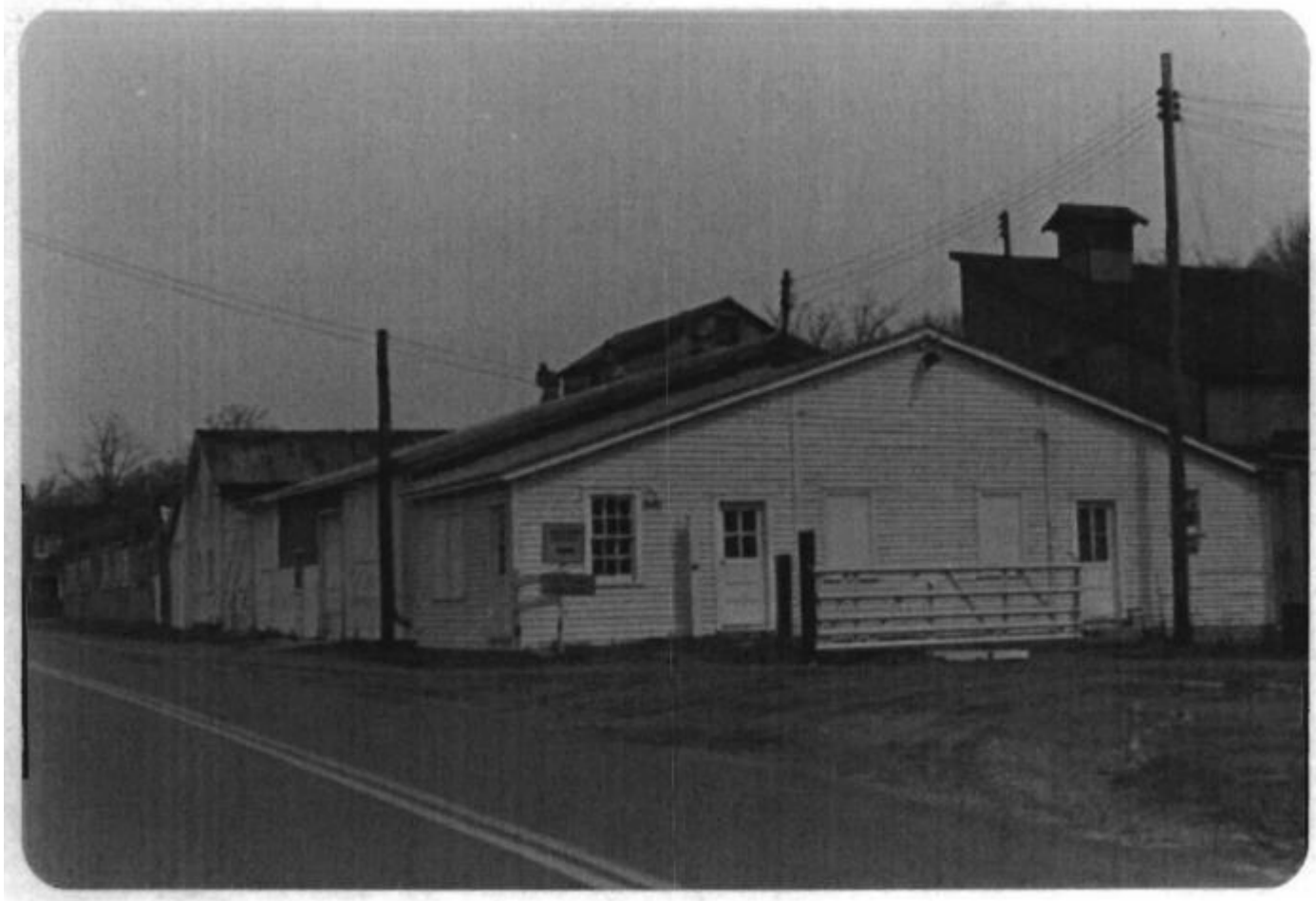
Figure 31. The Former Bottling Plant in 1981, looking northeast from Laird Road. The building volumes in the foreground have been demolished; the existing Former Bottling Plant buildings are situated in the background. (Source: New Jersey Historic Preservation Office.)
