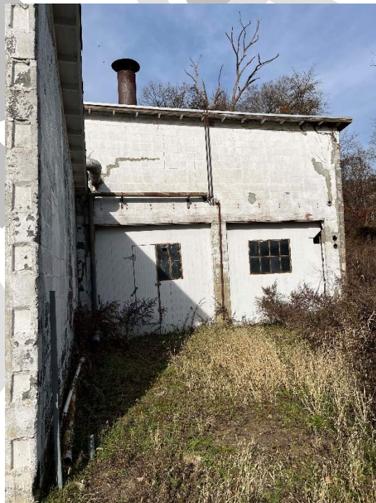
Photo 36. Exterior view of the Still House attached distillery equipment rooms, Volume D south (primary) façade, camera facing north (November 17, 2023).
