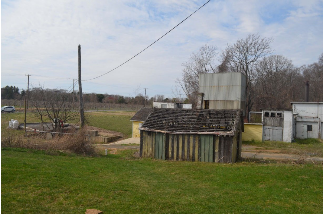
Figure 34. Exterior view of the Office prior to the roof's collapse, south elevation, within the surrounding context of the distillery complex, camera facing northwest (April 11, 2019).
