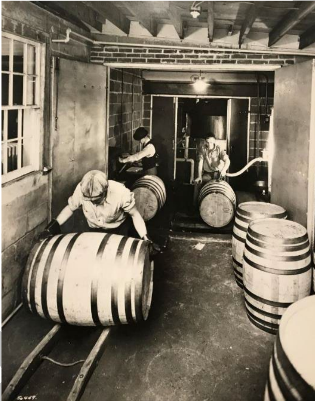
Figure 17. Preparing applejack barrels, interior of an unspecified building at the distillery, 1935. (Source: Laird & Company Archive.)
