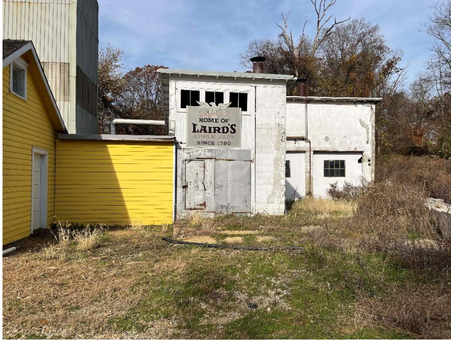
Photo 35. Exterior view of the Still House (right) attached distillery equipment rooms, Volumes B, C, and D, camera facing north (November 17, 2023).
