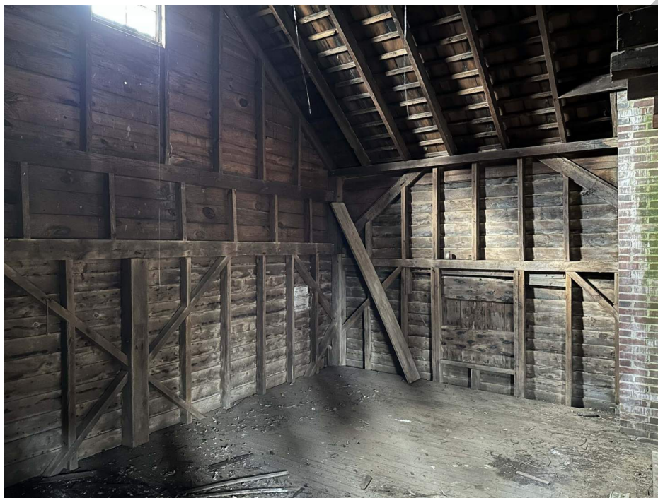
Photo 25. Interior view of the Barn, northwest corner of the second floor in Volume C. Interior of north and west elevations and exposed roof structure, indicating two different phases of construction. Camera facing northwest (November 17, 2023).
