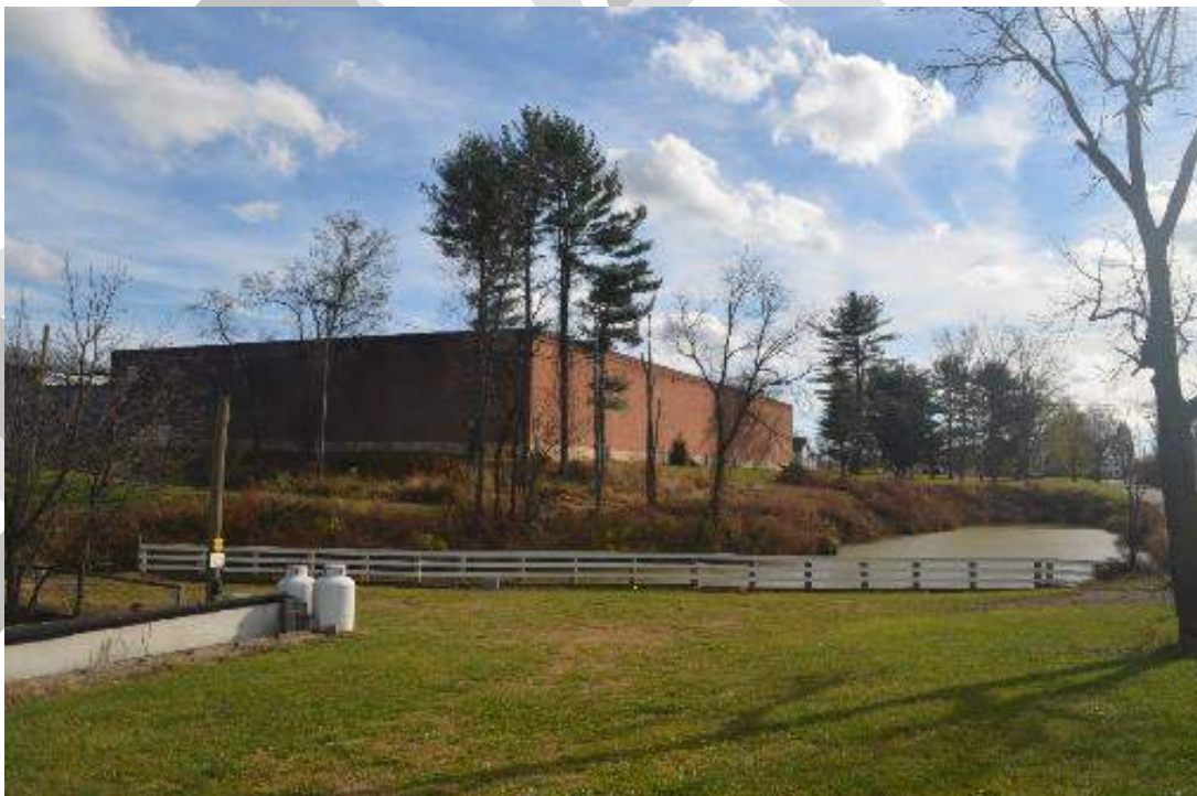
Photo 4. View of the Current Bottling Plant and dam (left), and man-made pond (right), camera facing south (November 17, 2023).
