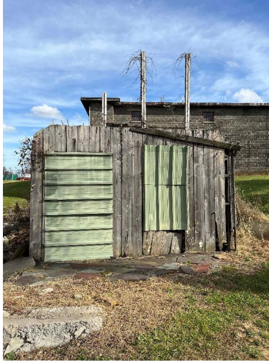
Photo 27. Exterior view of the Office, west (primary) façade, camera facing east (November 17, 2023).
