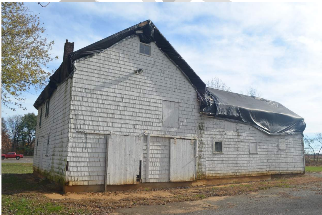
Photo 14. Exterior view of the Barn, west elevation, camera facing southeast (November 17, 2023).
