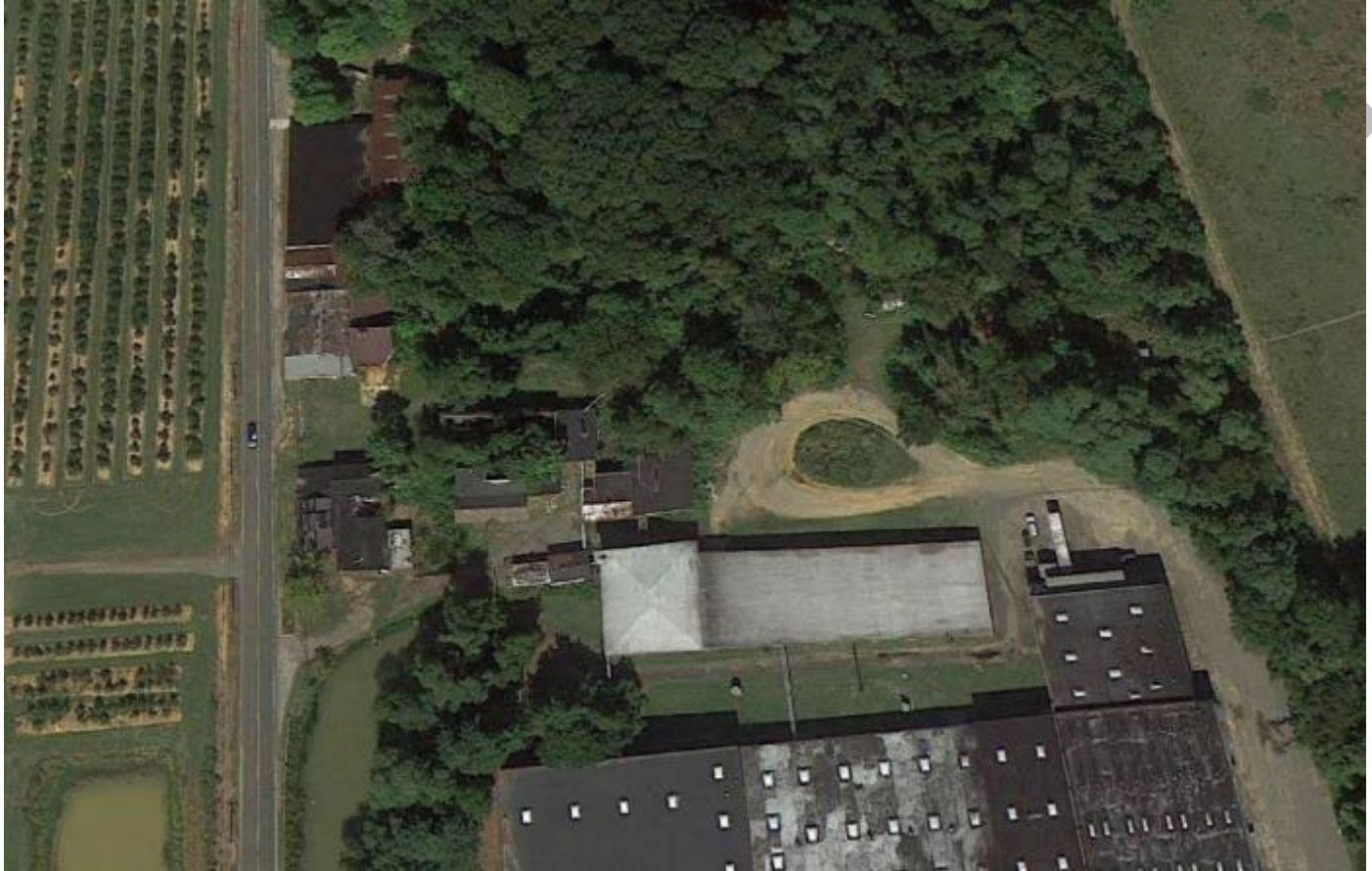
Figure 33. Aerial photograph from 2010 that captures the full distillery complex layout prior to the demolition of several former distillery buildings. The Former Bottling Plant is situated at the top left, the dam and pond at lower left, and the Still House, Office, and Bonded Warehouse are at center. (Source: Google Earth.)
