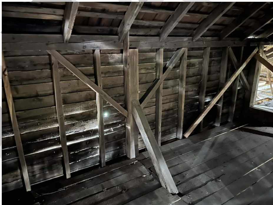
Photo 24. Interior view of the Barn, exposed wall and roof framing in the middle section of the Barn (Volume B) at the interior side of the east elevation, camera facing east (November 17, 2023).
