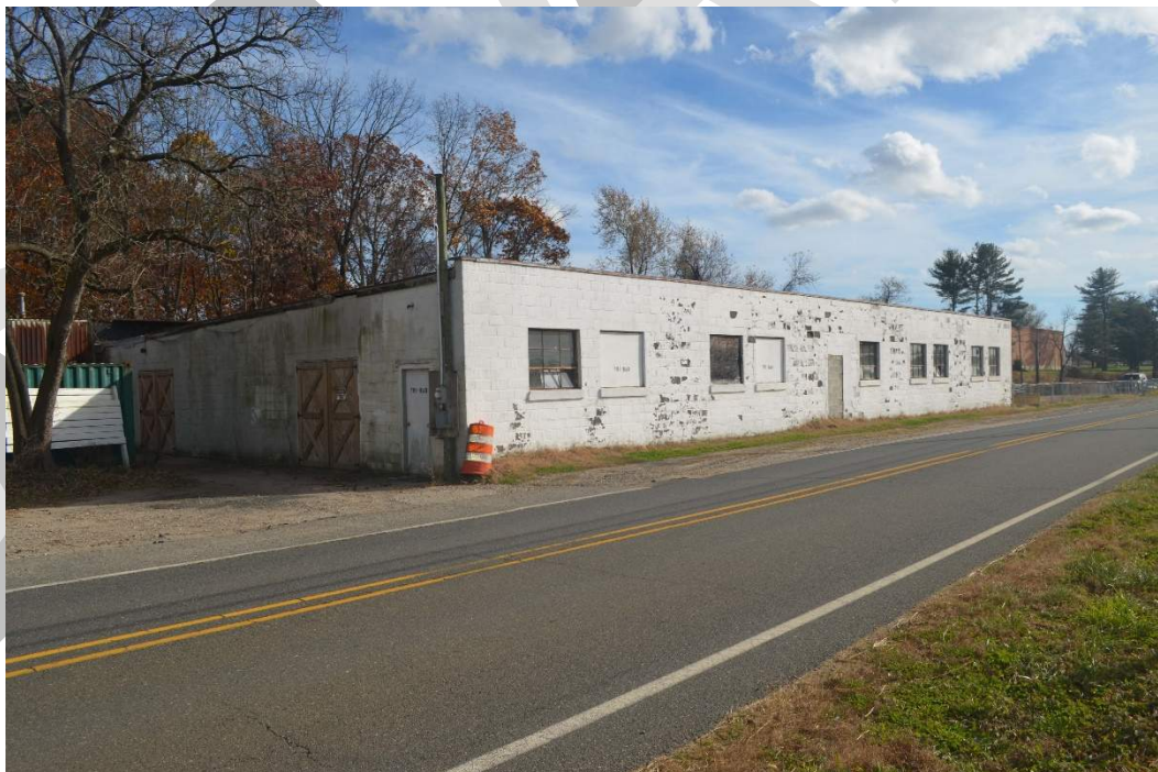
Photo 42. Exterior view of the Former Bottling Plant, north and west elevations of Volume A, camera facing southeast (November 17, 2023).
