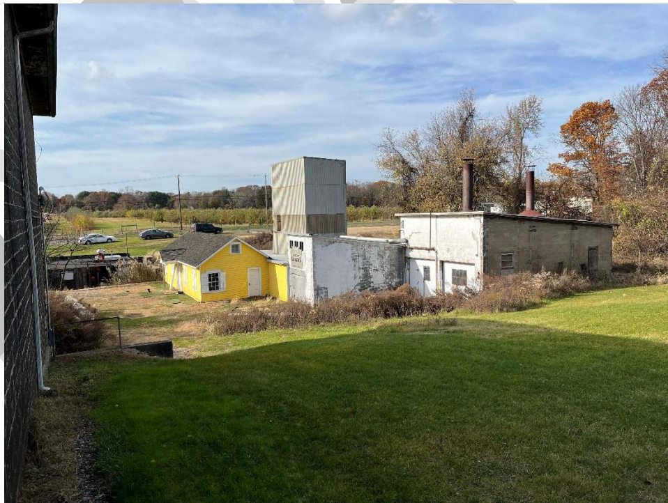
Photo 34. Exterior view of the Still House (left) and attached distillery equipment rooms, camera facing northwest (November 17, 2023).
