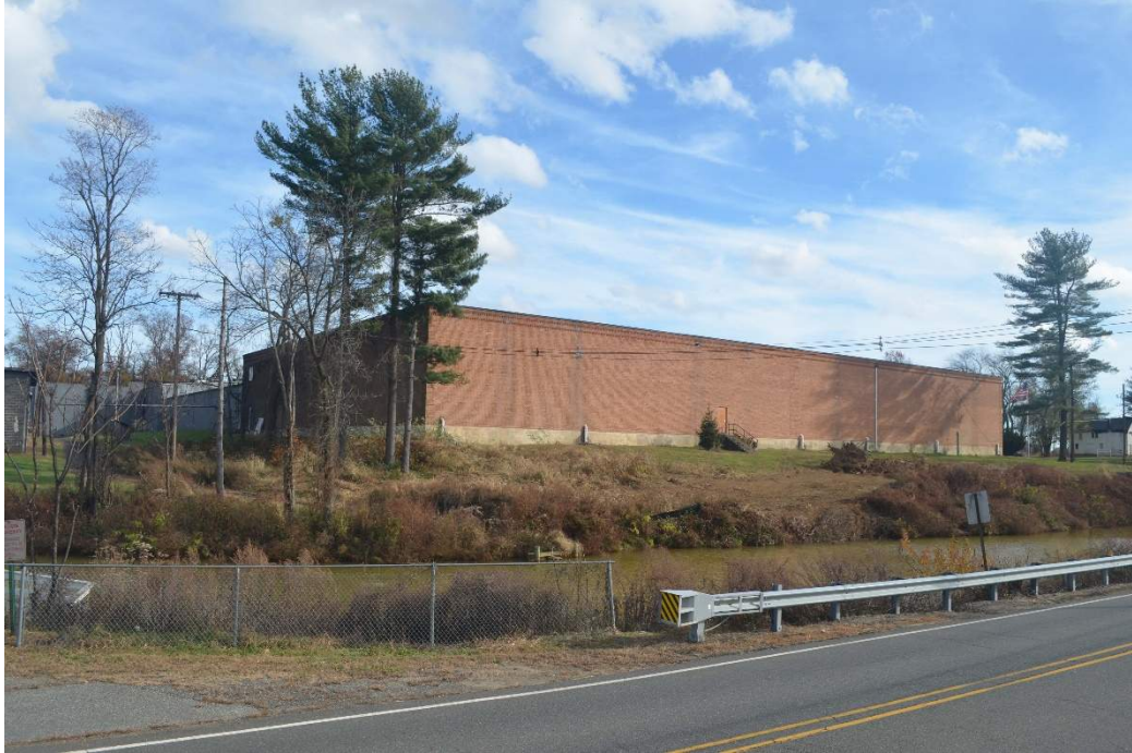
Photo 55. Exterior view of the Current Bottling Plant, north and west elevations, camera facing southeast (November 17, 2023).
