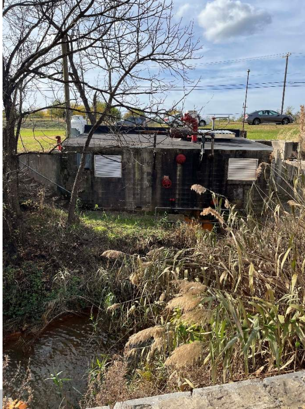
Photo 63. Exterior view of the Mechanical Equipment Shed built into the dam, camera facing west (November 17, 2023).
