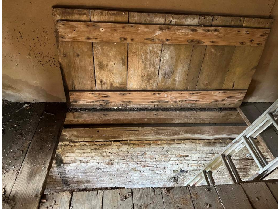
Photo 17. Interior view of the Barn, southernmost room of the first floor in Volume A, the oldest section of the Barn, with opening to root cellar, camera facing west (November 17, 2023).
