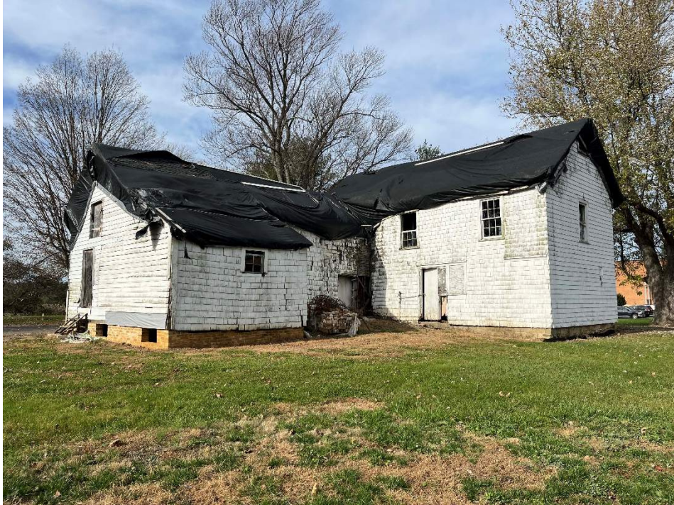
Photo 15. Exterior view of the Barn, east and south elevations, camera facing northwest (November 17, 2023).
