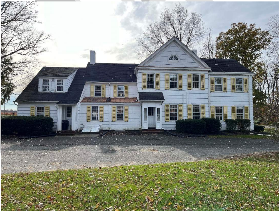
Photo 6. Exterior view of the House, north (rear) elevation, camera facing south (November 17, 2023).
