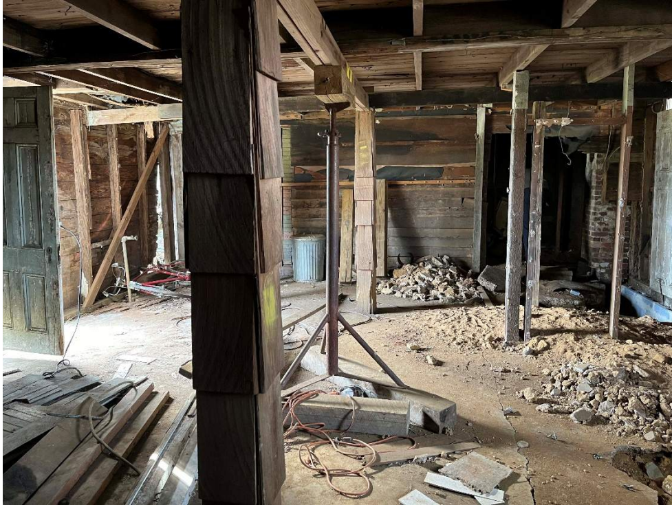
Photo 21. Interior view of the Barn, northwest room of the first floor in the north section of the Barn, Volume C, camera facing west (November 17, 2023).
