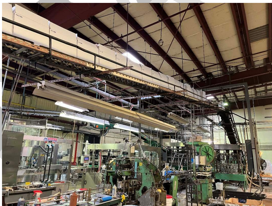
Photo 60. Interior view of the Current Bottling Plant, bottling equipment with conveyor belts carrying boxed bottles over the machinery, camera facing southeast (November 17, 2023).
