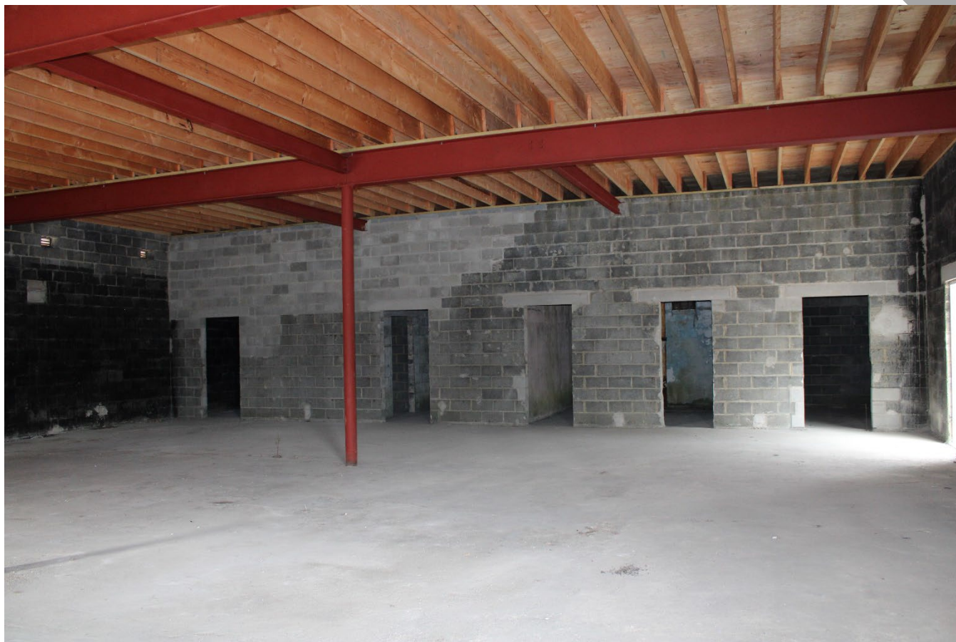
Photo 0003: View of the interior looking at the main space in the foreground and the doors to the support spaces in the rear ground, camera facing southwest.
