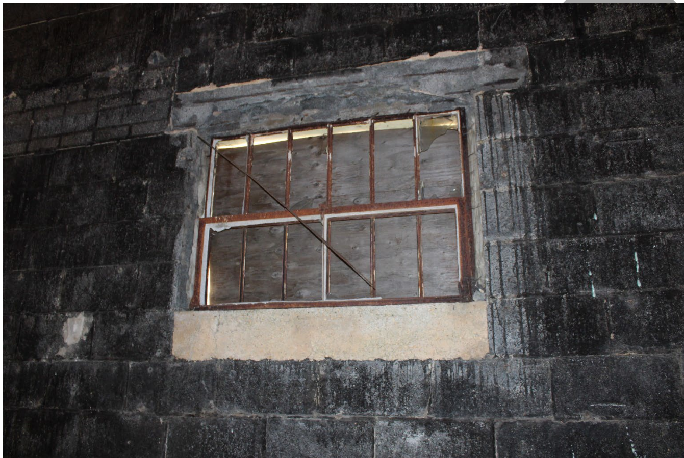
Photo 0005: View of a typical hot-rolled steel window showing lower two-light interior hopper with outer six-over-six exterior sash; camera facing east.
