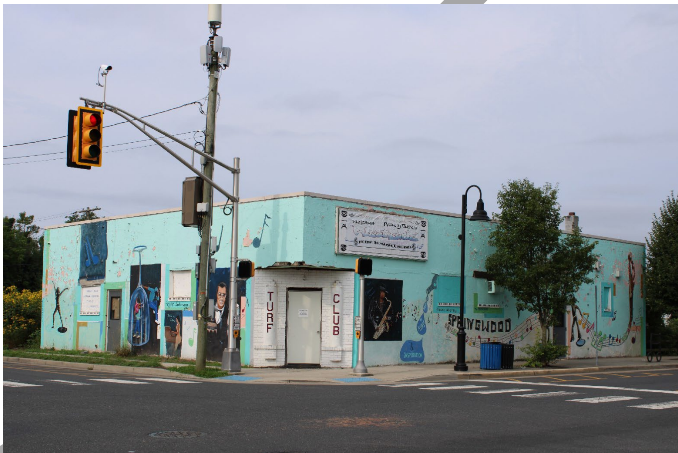
Photo 0001: Overall view of the Turf Club looking at the north and east street-facing elevations; camera facing southwest.
