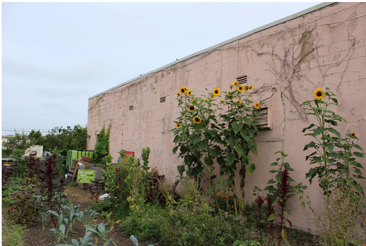
Photo 0012: View of the south elevation showing an unadorned façade, camera facing northwest.
