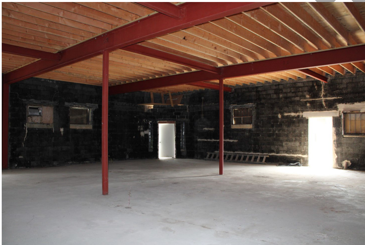
Photo 0016: View of the interior looking at the fenestration in the main space, camera facing northeast.
