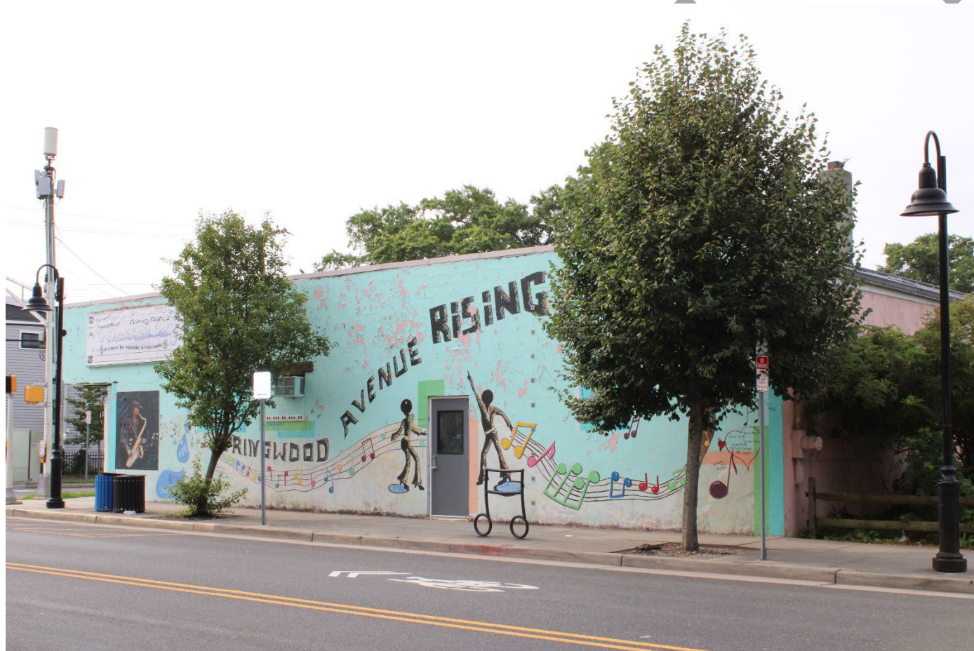
Photo 0007: View of the north elevation; camera facing southeast.
