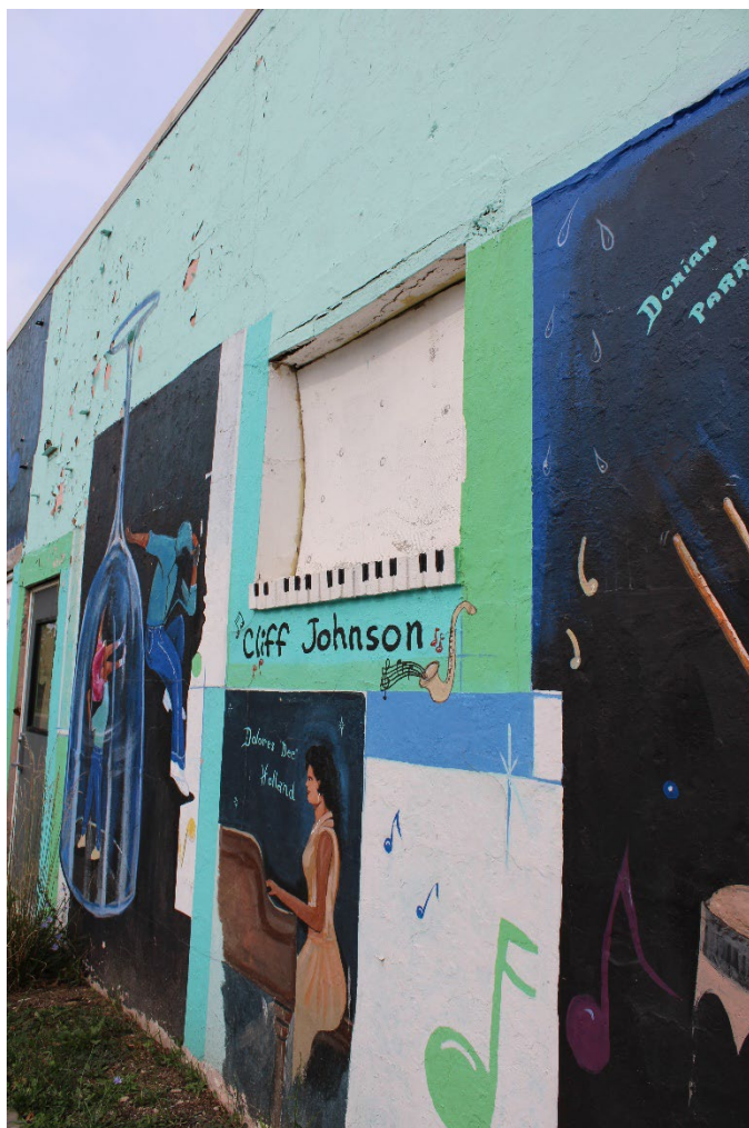
Photo 0006: Detail view of a window opening showing the projecting brick sills and plywood in front of the steel windows, camera facing south.
