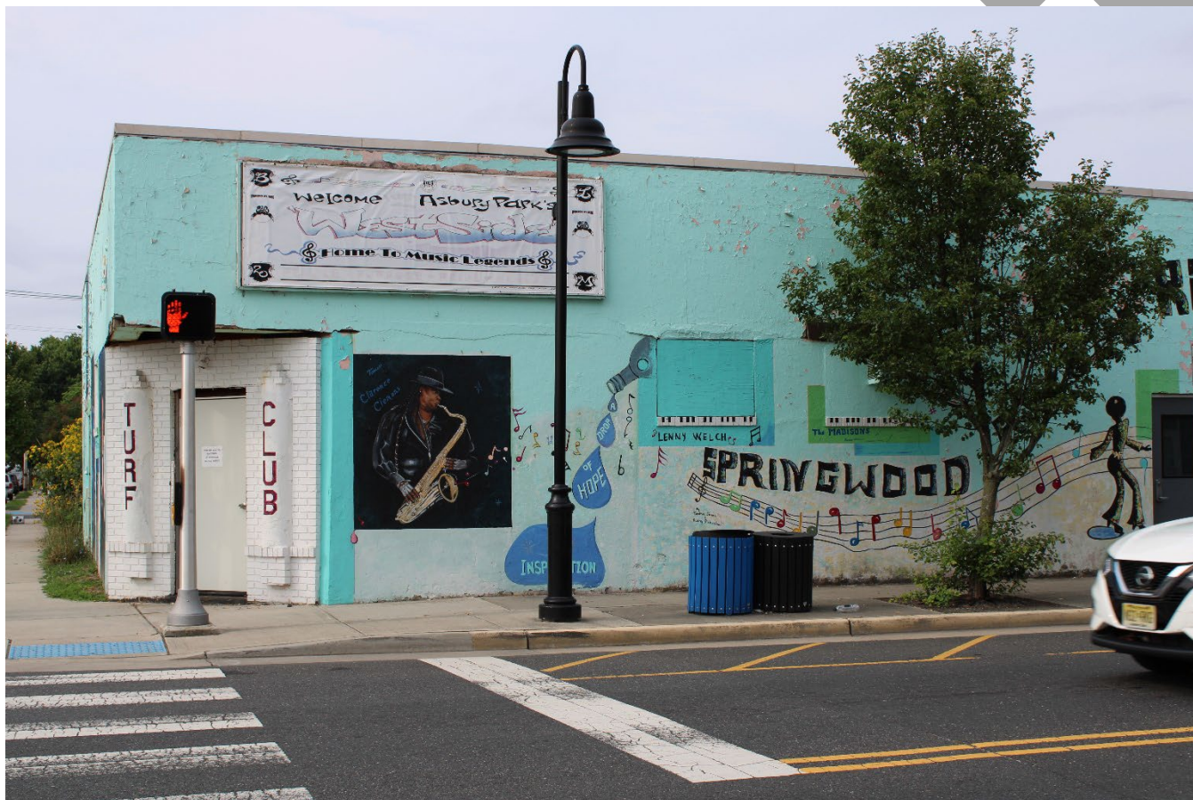
Photo 0004: View of the exterior looking at the north elevation showing the fenestration, signage, and contemporary mural, camera facing south.
