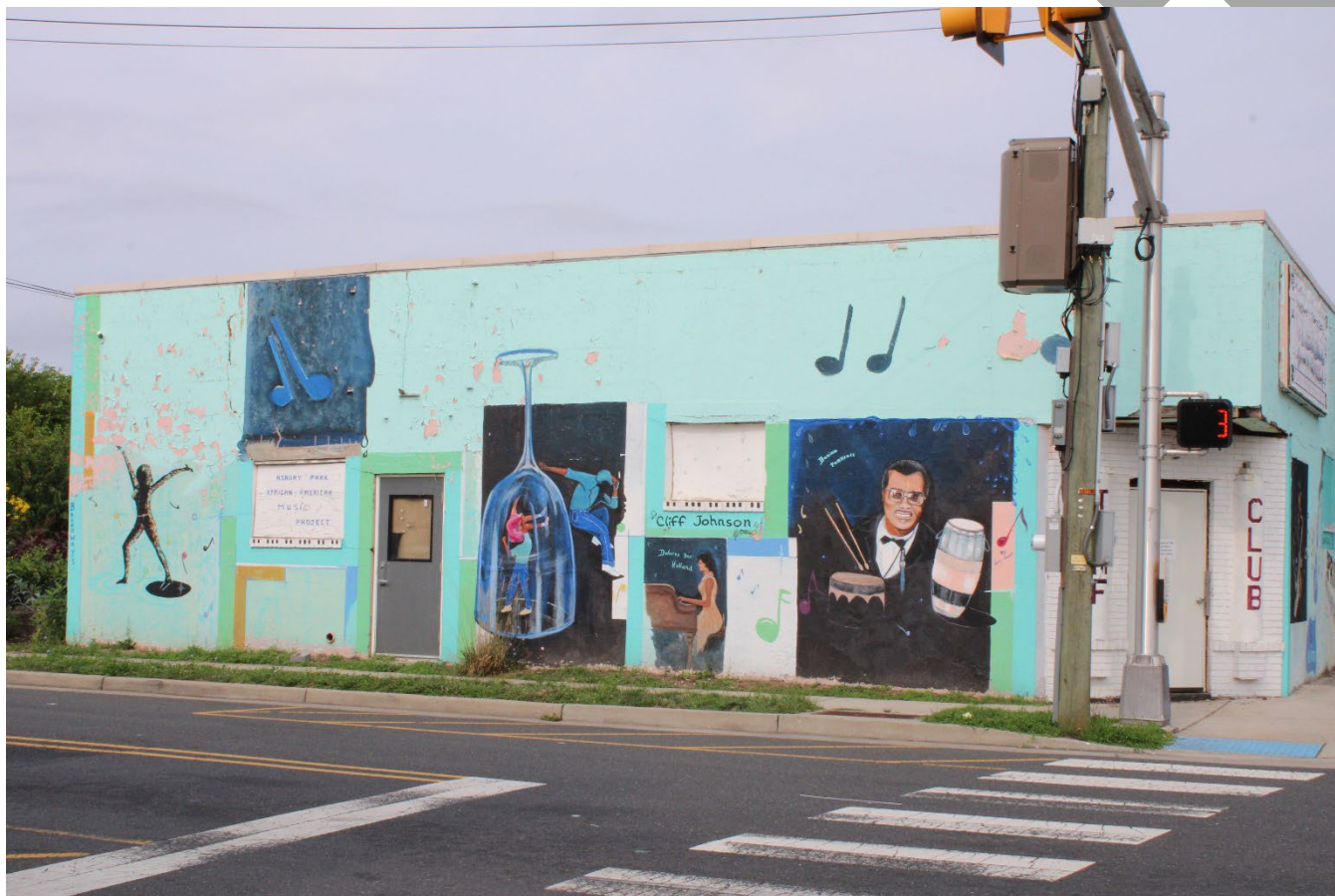
Photo 0010: View of the east elevation; camera facing west.
