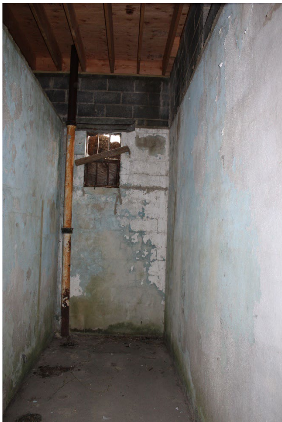
Photo 0018: View of one of the center support spaces along the west side of the building showing some of the remaining plaster finishes and the multi-light hopper steel window, camera facing west.
