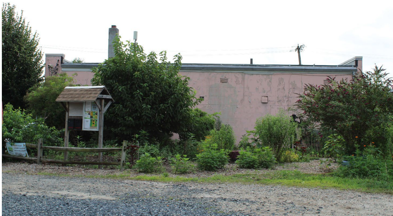
Photo 0014: View of the west elevation, which has minimal fenestration and is unadorned, camera facing east.
