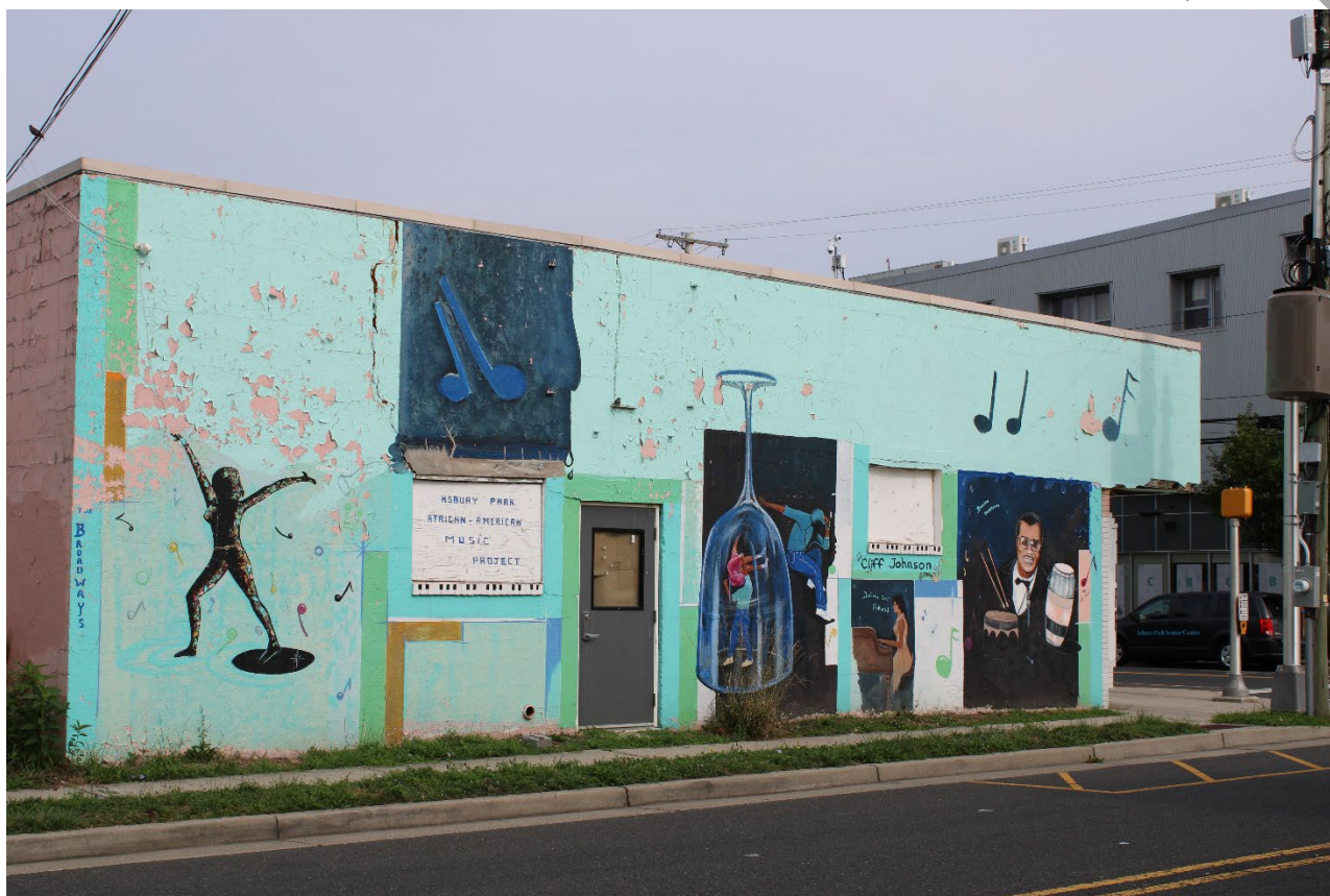
Photo 0011: View of the east elevation showing the minimal fenestration and contemporary mural camera facing northwest.
