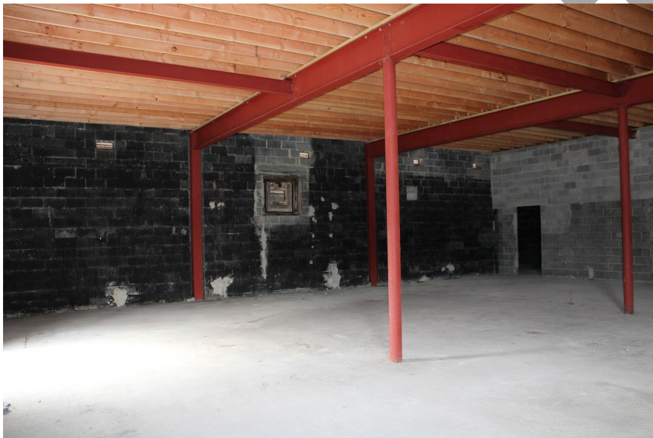
Photo 0015: View of the main space at the interior focusing on the east exterior wall and shows the original steel structure, camera facing southeast.
