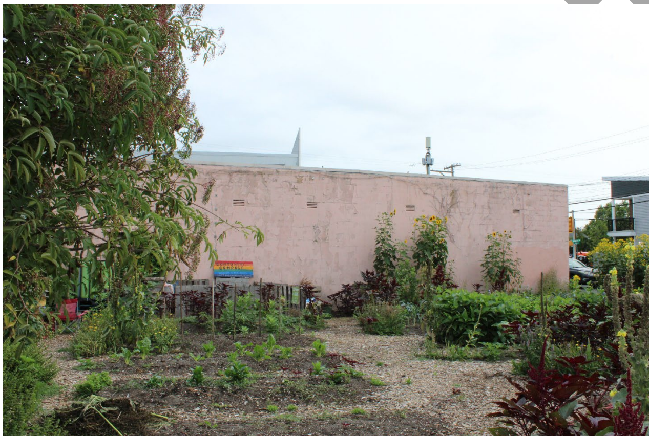
Photo 0013: View of the south elevation showing the unadorned façade meant to stand next to other buildings, camera facing north.
