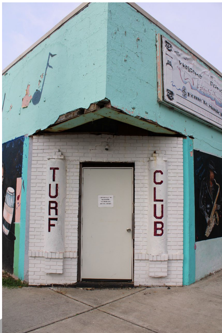
Photo 0002: View of the main entrance to the Turf Club looking at the clipped entrance at the corner of Springwood and Atkins Avenues, camera facing southwest.
