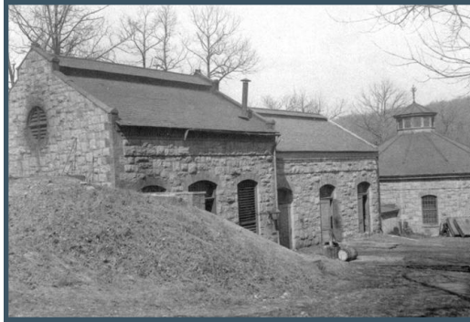
HISTORIC VIEW OF ORIGINAL GASHOLDER AND 1876 RETORT/PURIFICATION HOUSE C. 1890 GREYSTONE SCRAPBOOK
