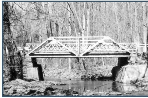
PECK'S FERRY BRIDGE HUNTERDON COUNTY
