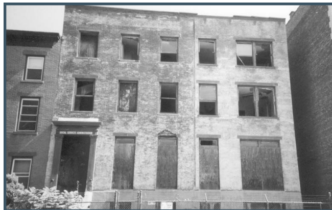
Located within the Van Vorst Park National Register Historic District, this vacant building is one of many in Jersey City that is being rehabilitated with an Investments Tax Credit. Photo by Gerry Bakirtjy, Architect.
