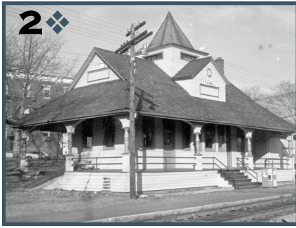
2 ORADELL RAILROAD STATION REHABILITATION, ORADELL BOROUGH, BERGEN COUNTY
