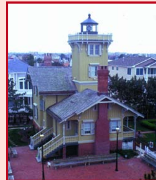
Hereford Inlet Light Station, North Wildwood, Cape May County, for restoration.
