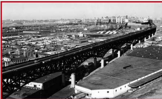
Photo from the Historic American Engineering Record. View of Pulaski Skyway over the Passaic River, looking into NYC – Jack Boucher, photographer, 1978
