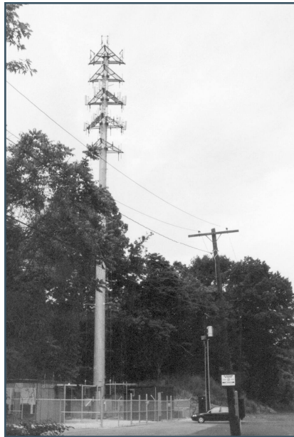
Example of a monopole with five co-located carriers
