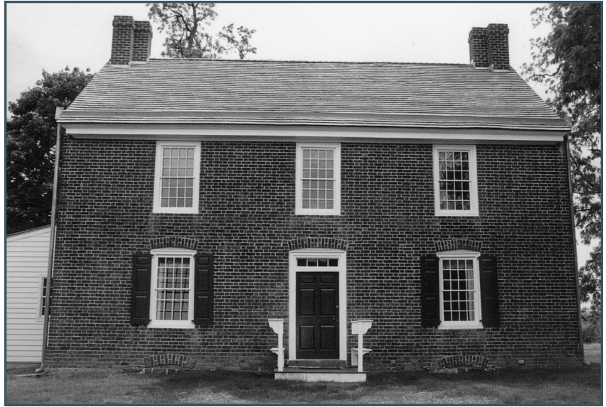
The application of the Rehabilitation Subcode allowed substantially more of the historic fabric and spaces of the Brearley House in Lawrenceville to be preserved than would have been possible under previous codes. Under the Rehabilitation Subcode, the open central stair was allowed to remain – the enclosure of the stair which was required by prior codes was not required. The existing plaster on lath walls were also accepted as a sufficient fire barrier to separate the caretakers quarters and the museum, thus allowing preservation of the existing walls and finishes.
