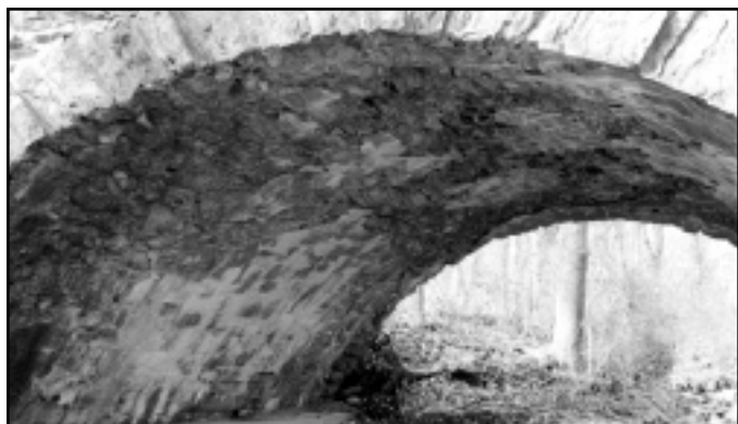
PALATINE ROAD BRIDGE, TEWKSBURY TOWNSHIP
