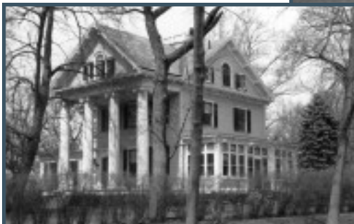
LIVINGSTON HOMESTEAD, HIGHLAND PARK
