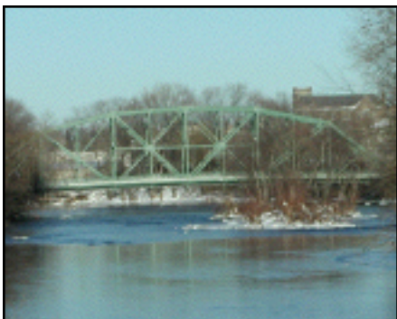
Straight Street Bridge Rehabilitation
