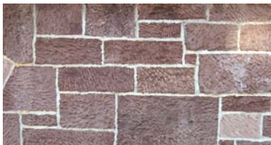
Figure 1. Brownstone construction detail, Geology Museum, Rutgers University, New Brunswick, Middlesex County. Photo by Z. Allen-Lafayette
