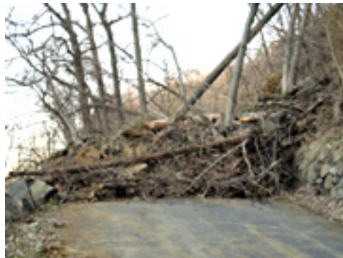
Figure 5. Landslide blocks Henry Hudson Drive. Photograph courtesy of Palisades Interstate Park - NJ Section
