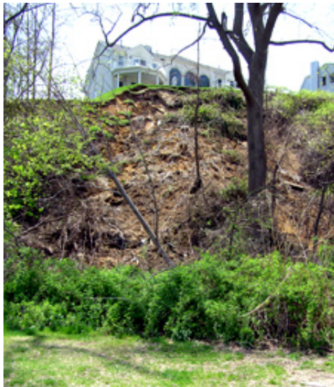
Figure 4. Highlands Boro landslide. Photo by S.D. Stanford
