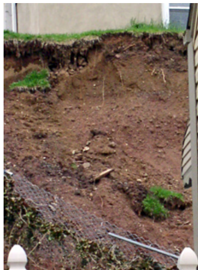
Figure 2. One of the four Farnham Avenue landslides. Photo by T. Pallis
