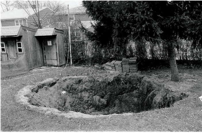
Figure 1. Collapse in North Arlington Boro, Bergen County. Photo courtesy Borough of North Arlington
