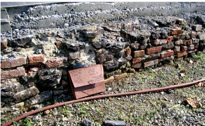
Figure 4. Steam engine and boiler house wall built circa 1851. Note wall made of various sized bricks, purple red "Jersey" stone and recent cement floor overlying it. Photo by S.W. Johnson
