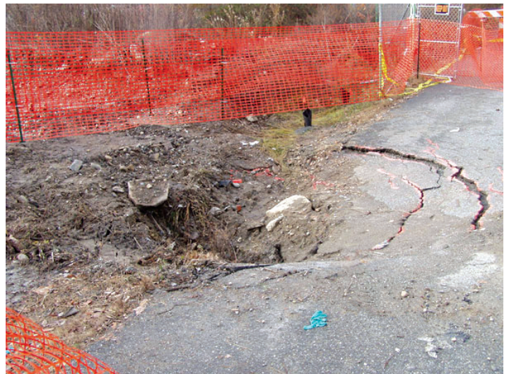
Figure 3. This collapse occurred where the road crossed the Cooper Mine. It is approximately 125 feet from a previous collapse in the back yard of a private home, Ringwood Boro, Passaic County. Photo by R.A. Volkert
