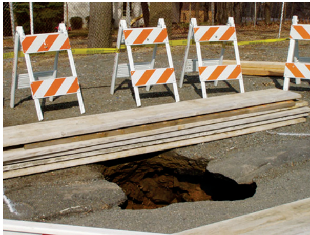
Figure 2. Collapse along the White Meadow Mine workings, Rockaway Twp, Morris County. Photo by R.A. Volkert
