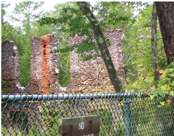
Figure 5. A portion of the Paper Mill's west wall today. Small amounts of white stucco remain on the wall from the original finished surface. Photo by S.W. Johnson.
