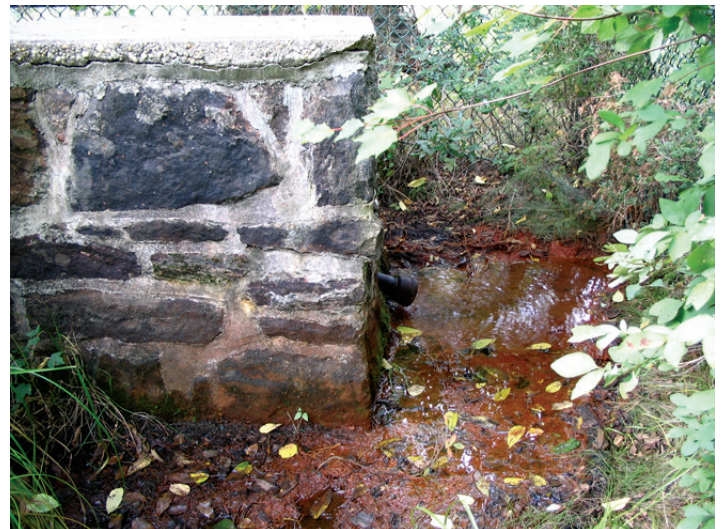
Figure 1. R.C. Harris Well, Harrisville, Burlington County. Note orangey brown stains (caused by precipitation of iron) near discharge pipe. The flow varies seasonally from 5-10 gallons per minute with lows in late summer and fall and highs in winter and spring. Photo by S.W. Johnson
