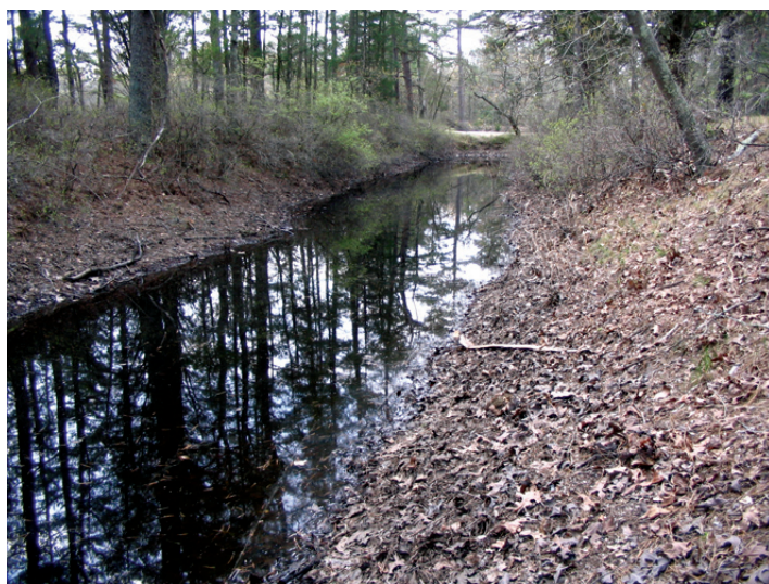
Figure 3. Harrisville Canal constructed in the 1830's by McCarty's Wading River Manufacturing and Canal Company and modified in the 1860's by Harris. Canal conveyed impounded water to the turbines which powered the paper mill. Canal in this view is approximately 25 feet wide by 8-10 feet deep. Photo by S.W. Johnson.
