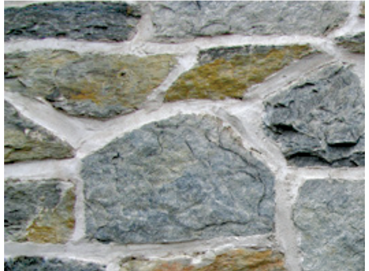
Figure 4. Close-up of exterior wall of barracks showing blocks of quartz-sericite schist (light gray) and blue quartz-pebble conglomerate (dark gray) of the Chickies Quartzite. Photo by R.A. Volkert
