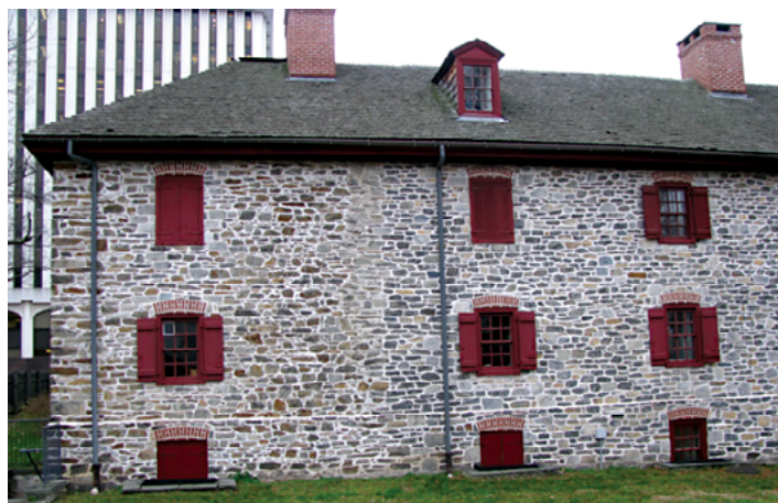
Figure 1. Rear view of the Trenton Barracks, showing original stonework, left, and restored stonework from 1915-1916, right. Photo by R.A. Volkert
