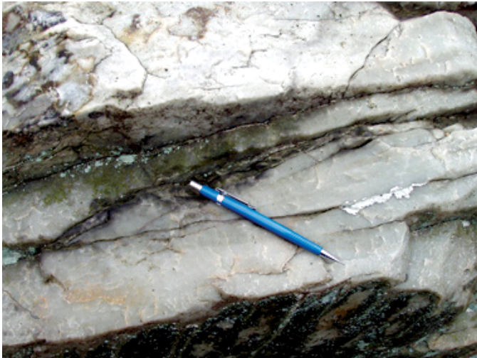
Figure 4. Close-up of exterior wall of barracks showing blocks of quartz-sericite schist (light gray) and blue quartz-pebble conglomerate (dark gray) of the Chickies Quartzite. Photo by R.A. Volkert
