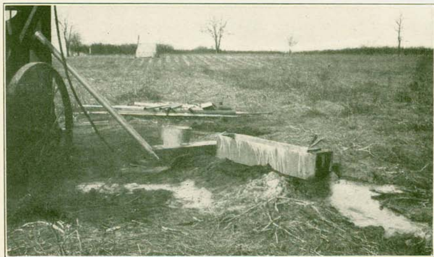
B. SAMPLING TROUGH IN USE AT ELMWOOD ROAD, BURLINGTON COUNTY, N. J.
