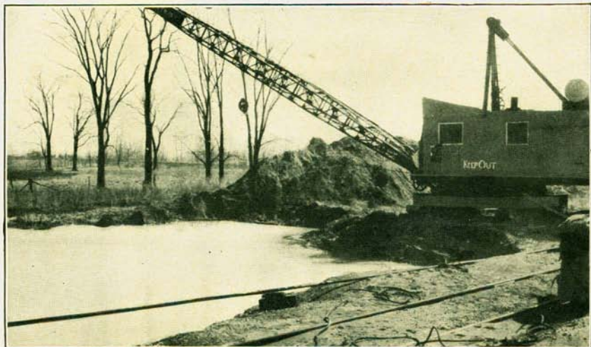
A. DREDGE, PIT, AND STOCK PILE OF ATLANTIC POTASH CORPORATION ABOUT 1.1 MILES EAST OF MARLTON, BURLINGTON COUNTY, N. J.
