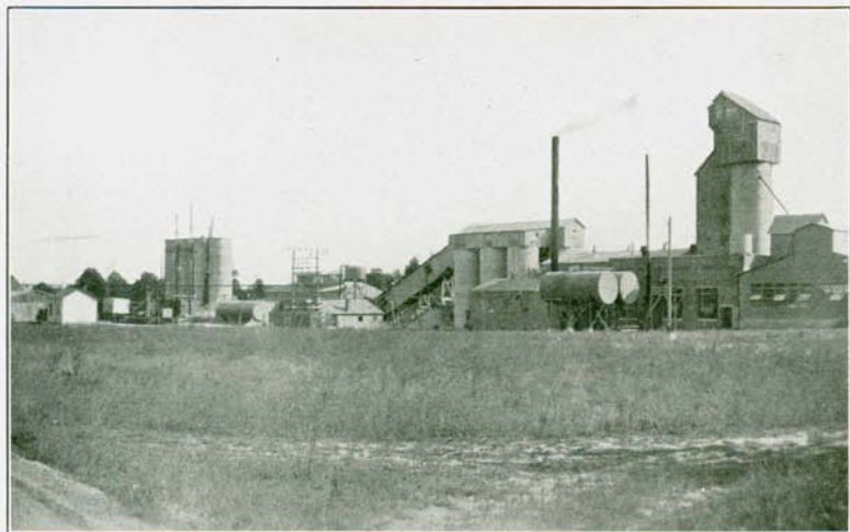
(a) Cleaning plant (left) of the South Jersey Sand Company. Storage and pulverizing plant of the Pennsylvania Pulverizing Company shown at right. Located near Dividing Creek Station, Cumberland County.
