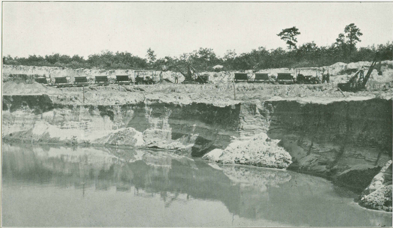
Sand pit near Manumuskin, Cumberland County. Well-bonded molding sand is dug from above the steep bank and carried in the cars shown to a railroad loading station. "Sharp" sand for foundry use is dug from the lower bank by a dredge operating in the pond shown.
