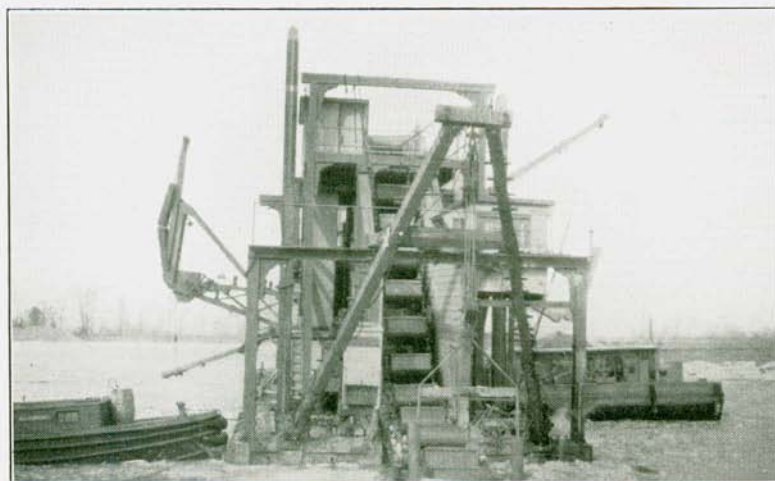
(b) River dredge operated by the Warner Company in Delaware River below Riverside, Burlington County.
