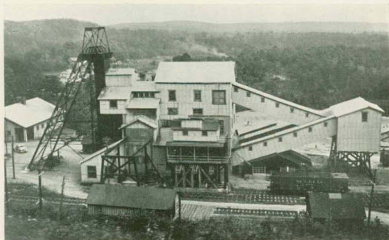
B. Mill and headframe at the Richard Mine of the Thomas Iron Company.
