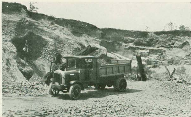
B. Small sand pit near Paterson. Note mechanical loaders and irregularity of deposits.
