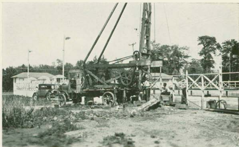
A. Drilling a well to supply pure water for a swimming pool near Princeton Junction. The rig is typical of the type commonly used to drill wells 50 to 1000 feet deep.
