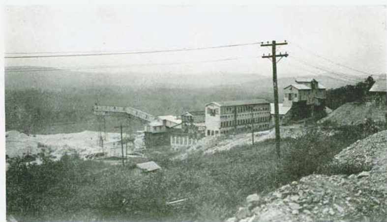
B. View to left of that above. Shows buildings which house crushing and screening equipment for reduction and sizing of rock waste, storage bins for ore concentrates, and tailings conveyor.
