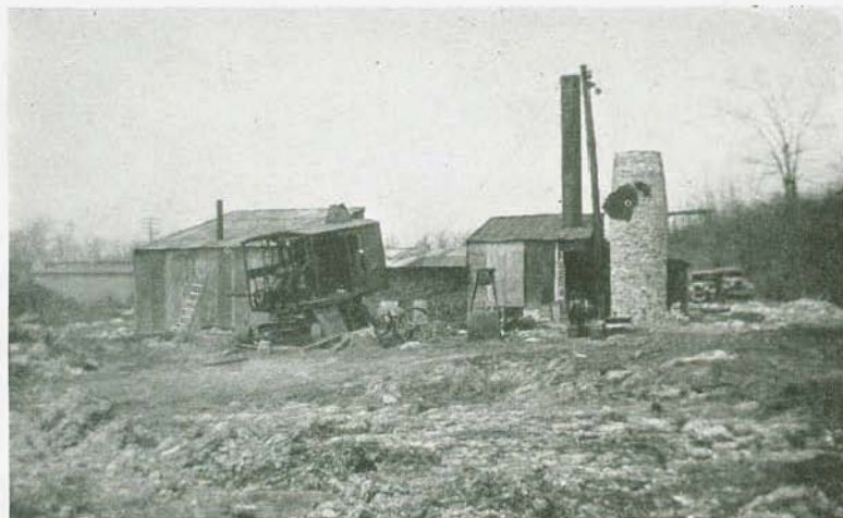
B. Plant erected by J. G. Marcrum to dry and pulverize the diatomaceous earth from a deposit just west of Lake Musconetcong.
