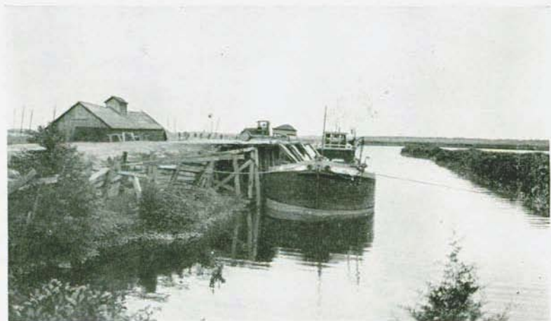
B. Shipping molding sand by barge from Dorchester, Cumberland County.
