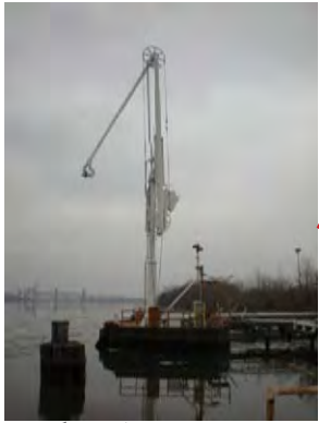
Loading Arm on Breasting Dolphin to load/unload ships.
