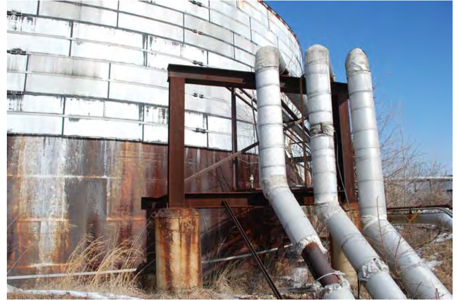
Above: Insulated tank with insulated pipe.
