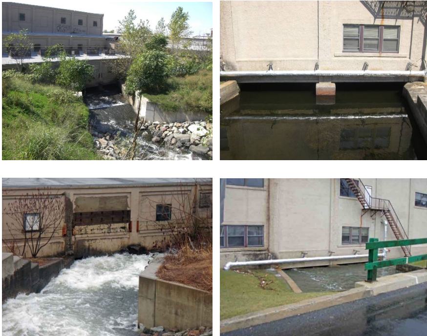
Old mill building across the Musconetcong River in Stanhope, low water (top) and high water (bottom)
