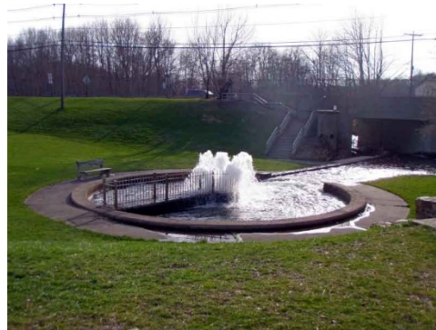
Fountain at Lake Hopatcong. Stream gauges are located under bridge in the background
