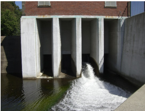
Lake Hopatcong sluice gates
