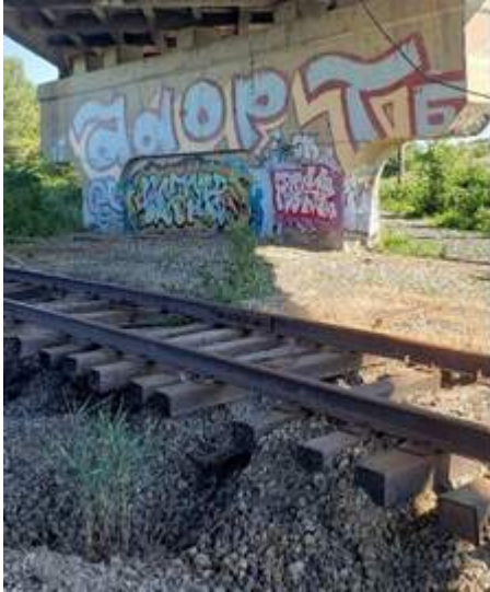
(5) The ground approximately 300 feet west of the bridge is washed out
