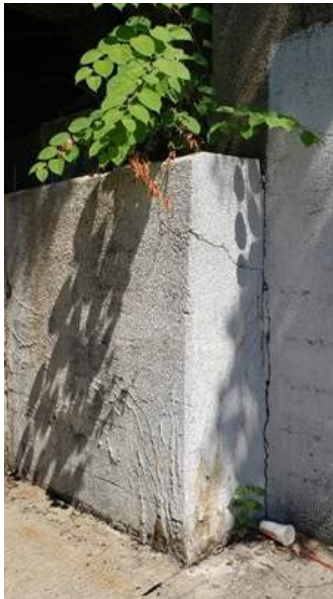
(9) East concrete abutment exhibiting some cracking
