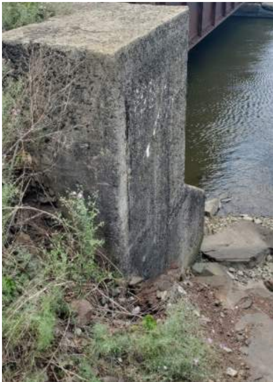
(11) View of east abutment with concrete in generally good condition
