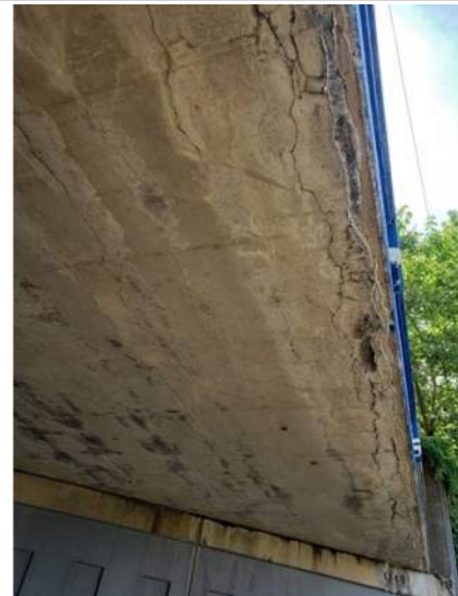
(6) Longitudinal cracking and spalling on underside of superstructure
