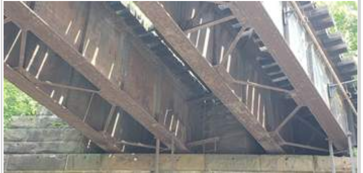
(6) Minor corrosion on the girders
