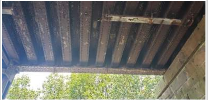
(4) View of underside of metal deck
