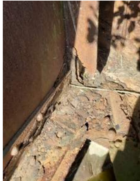
(6) Corrosion on the bottom flanges of the girders
