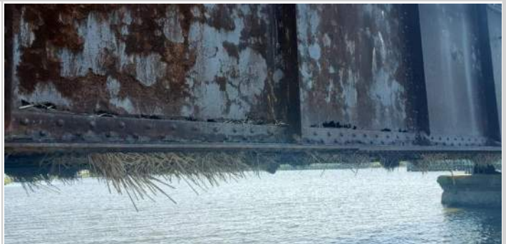
(6) Corrosion and section loss in bottom 1' of approach webs at southern girder west side
