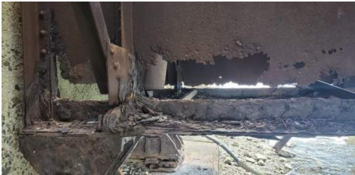
(9) Full section loss of web and severe deterioration of bottom flange in approach girders at east abutment
