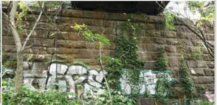
(2) West masonry abutment exhibiting some cracking
