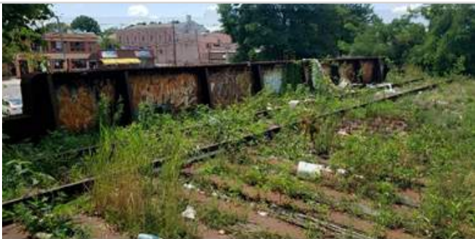
(7) View of overgrowth on top of metal deck
