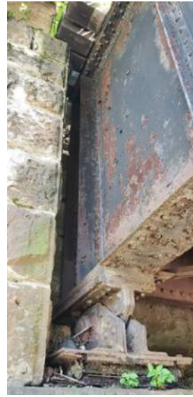
(8) Corrosion in girders and bearings
