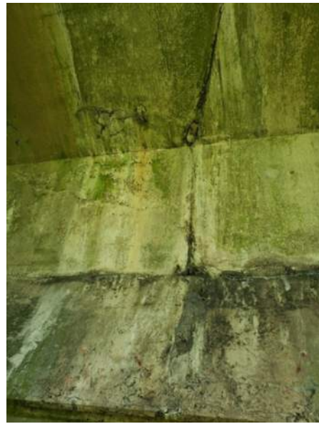
(12) Spalling and discoloration on the side of one of the piers
