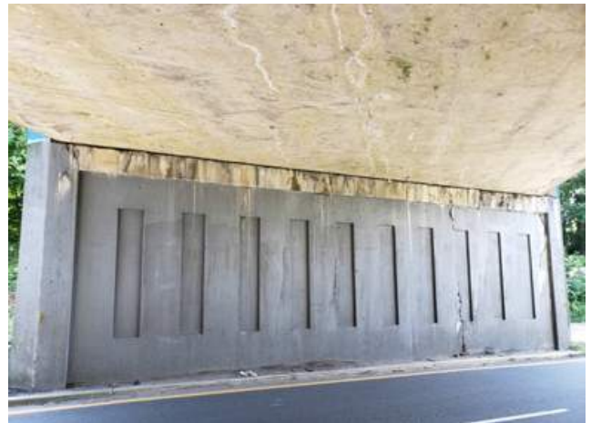
(8) Cracking on underside of deck and discoloration at the top of the pier
