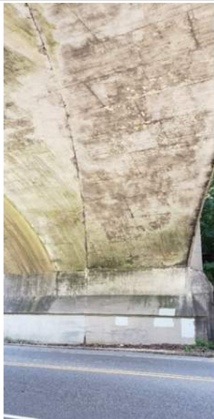
(9) Spalling at construction joint
