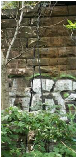
(3) West masonry abutment exhibiting some cracking
