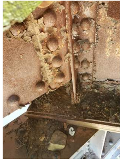
(6) Corrosion at a connection on the superstructure
