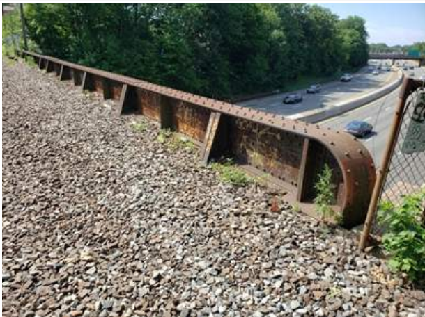
(3) Corrosion on the girder
