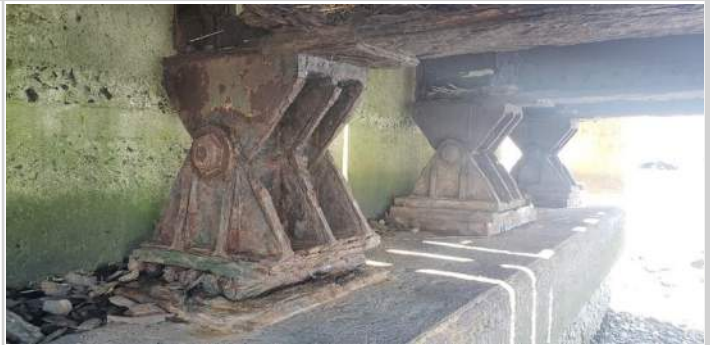
(4) Deterioration at bearings at west abutment
