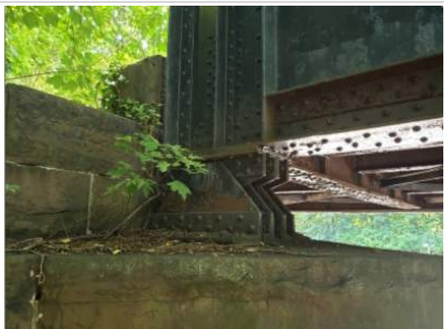
(4) Crack running horizontally in masonry under bearing
