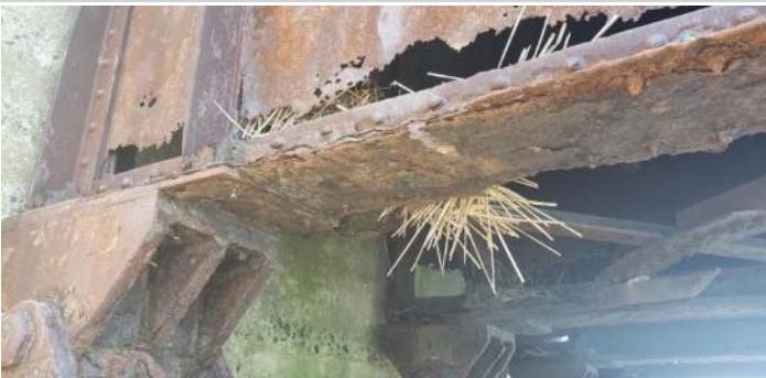
(5) 100% section loss in web and significant deterioration of bottom flange in approach girder at west abutment
