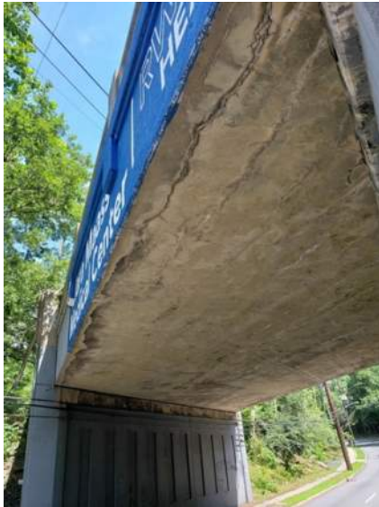
(7) Longitudinal cracking and spalling on underside of superstructure
