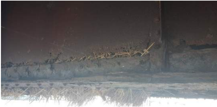
(7) Corrosion at section loss in bottom 1' of approach webs interior girder west side
