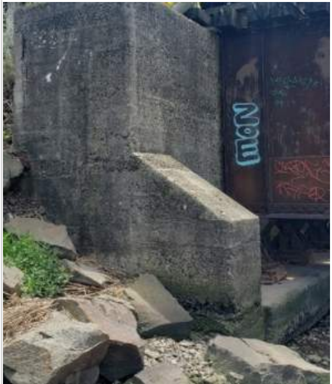
(12) View of east abutment, with concrete in generally good condition
