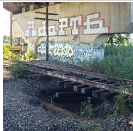
(4) The ground approximately 300 feet west of the bridge is washed out
