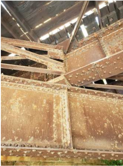
(3) Corrosion on superstructure
