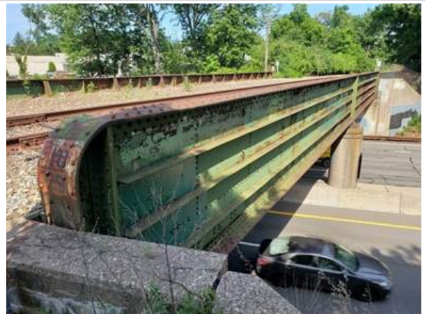
(6) Corrosion on the girders
