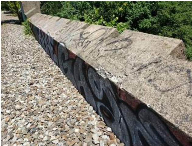
(3) Graffiti and some spalling on parapet
