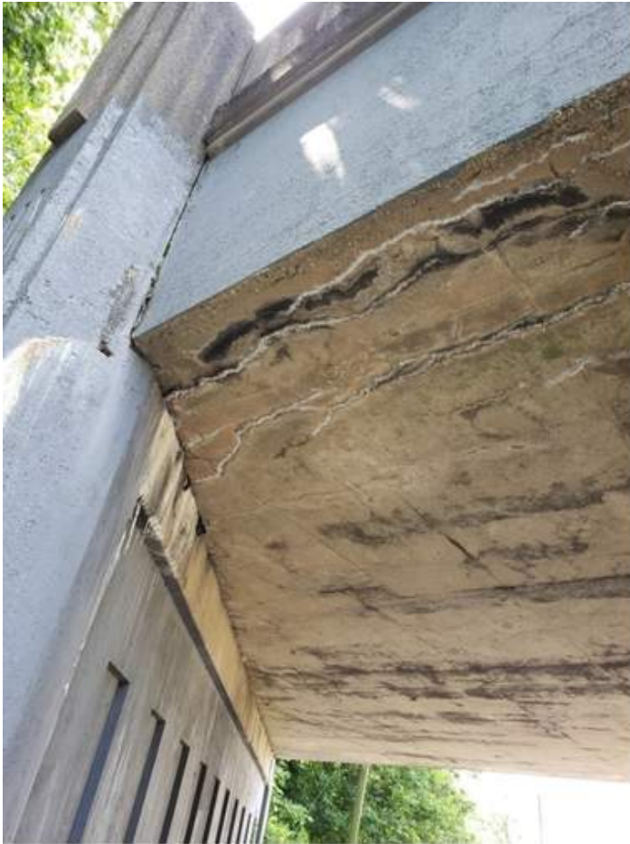
(11) Longitudinal cracking on underside of deck
