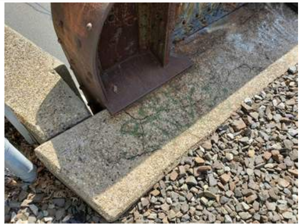
(4) Cracking in the concrete above the abutment
