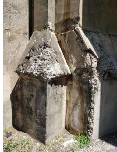
(8) Spalling at the base of one of the piers
