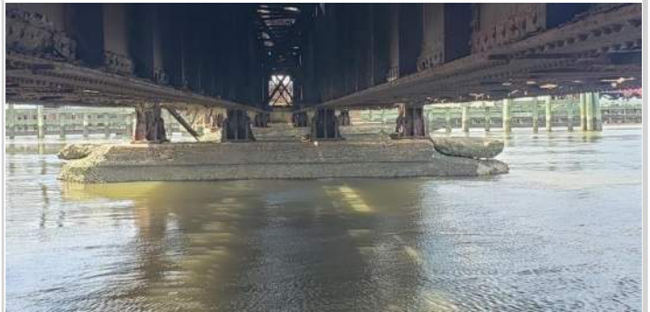
(10) Substructure in east approach with significant spalling at waterline
