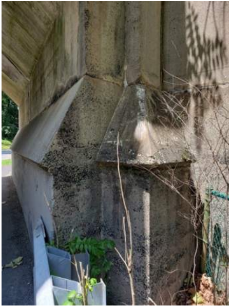
(11) Spalling at the base of one of the piers
