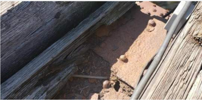
(3) Corrosion at top flange of approach girders between deck timbers
