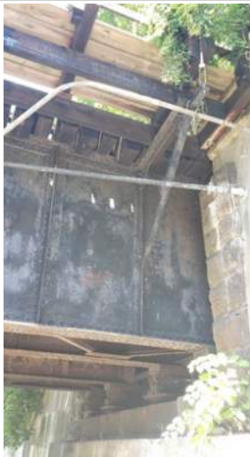
(5) Corrosion on the girders
