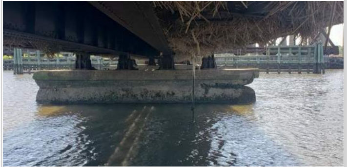
(8) View of spalling and section loss in substructure at waterline in west approach. Note sea grass stuck in girders
