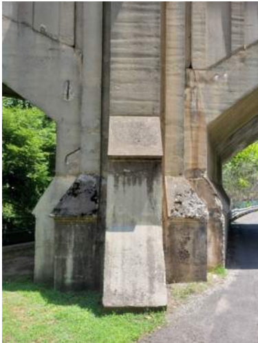
(7) Spalling at the base of one of the piers
