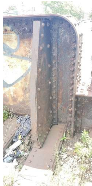
(6) Corrosion on one of the girders
