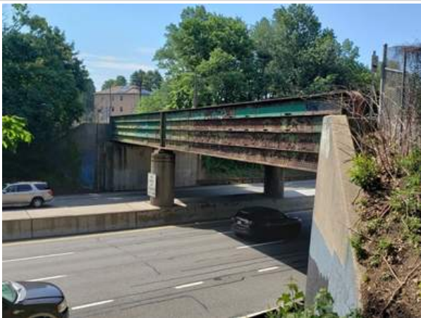
(5) Corrosion on the girders
