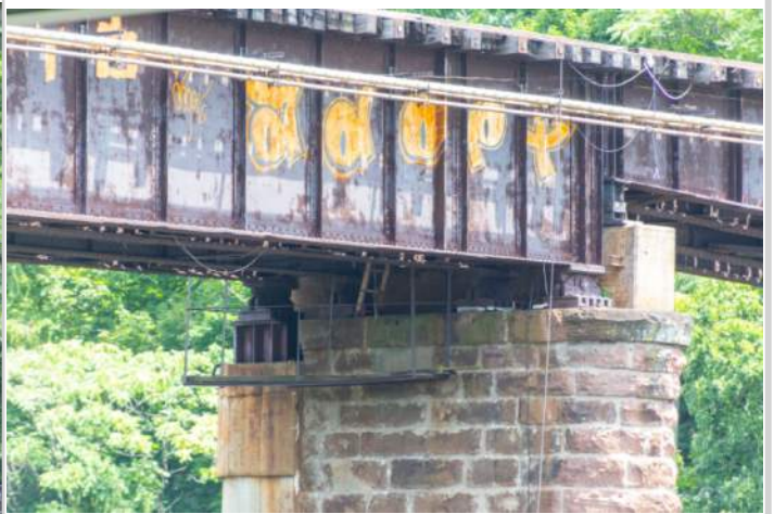
(12) Evidence of past rehabilitation measures used on the bearings at one of the piers
