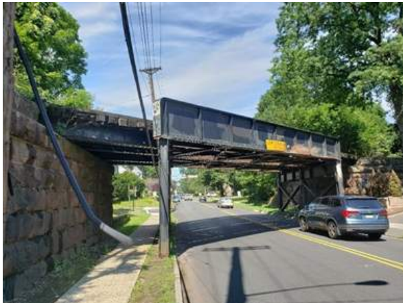
(1) Damage to the fascia girder due to vehicular impact
