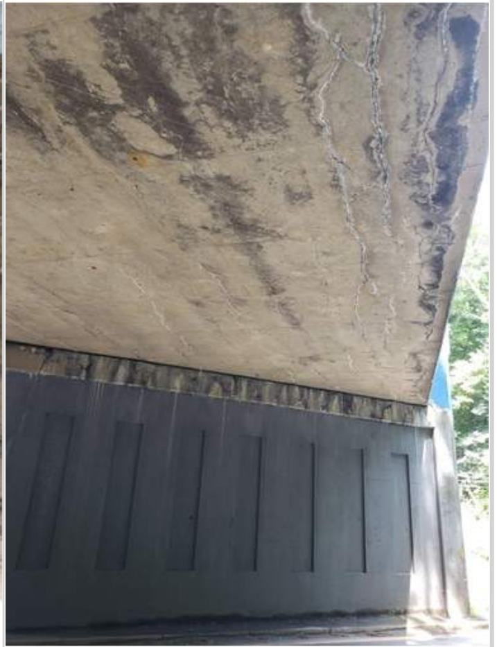
(12) Longitudinal cracking on underside of deck
