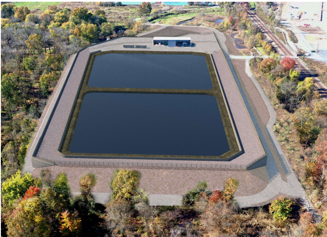
Rendered image of planned additional flood protection efforts surrounding Impoundments 1 and 2 looking west.
