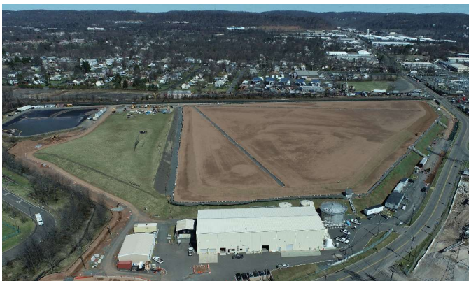
View of Impoundment 8 Facility Closure Looking North as of March 21, 2022
