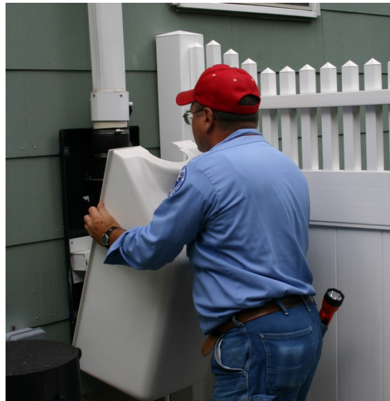
Figure 6-1 Inspection of SSD fan and weatherproof
