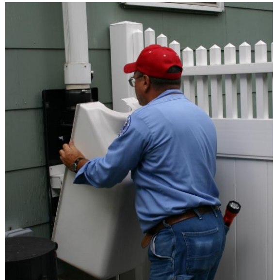
Figure 6-1. Inspection of SSD fan and weatherproof cover
