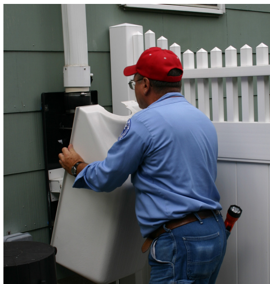
Figure 6-1. Inspection of SSD fan and weatherproof cover
