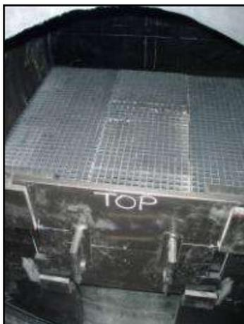
**Figure 3. Removable bulkhead door across from ingress/egress ladder at rear of filtration chamber.**
