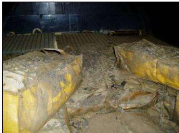
**Figure 4. Perlite filter media needs replacement.**
