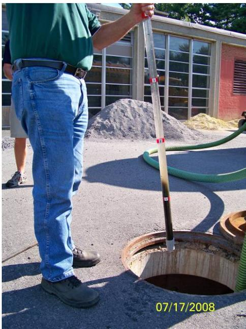
The depth of sediment and oil can be measured from the surface by using a sediment probe or dipstick tube equipped with a ball check valve and inserted through the Jellyfish Filter's maintenance access wall. The large opening in the maintenance access wall provides convenient access for inspection and vacuum removal of water and pollutants.
