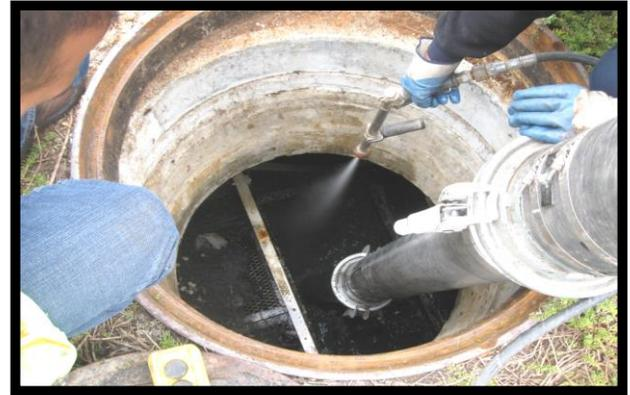
Insert Vacuum Hose in the Sedimentation Chamber and Vacuum Out All Trash, Sediment and Standing Water.
