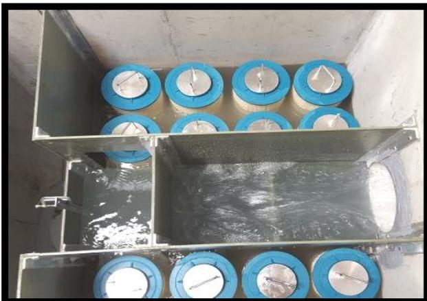
Assess the Condition of the Filter Cartridges and Determine If Cleaning is Required.
