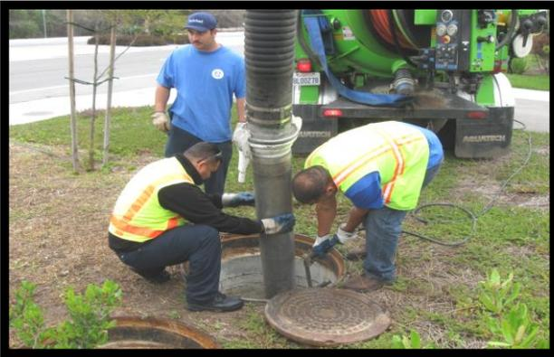
Remove Access Hatches Set Up Vacuum Truck to Clean The Pretreatment Chamber.
