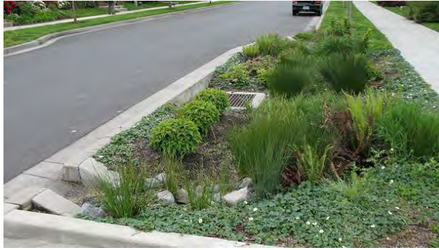
Figure 7.3: Example of a Green Street with incorporation of a Curb Extension and Rain Garden in Portland, OR 2
