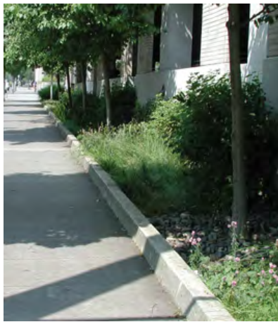
Figure 7.4: Example of a Green Street with incorporation of a flow-through planter in Portland, OR 2
