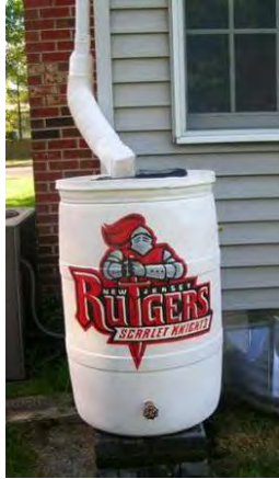
Figure 7.5: Example of an installed Rain Barrel in the Lower Delaware Watershed
