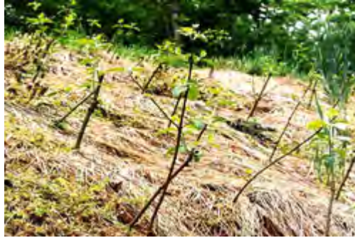
Figure 7.7: Erosion control and streambank stabilization with live stake plant material, North Carolina 3
