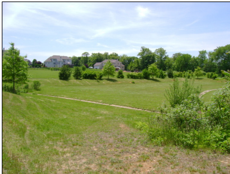
Figure 55. Dry detention basin at station #80, showing turf grass vegetation and concrete low-flow channels, photo taken in summer 2009.
