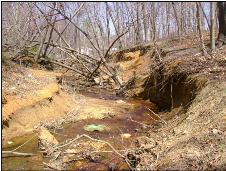
Figure 25. Station #29 looking downstream.
