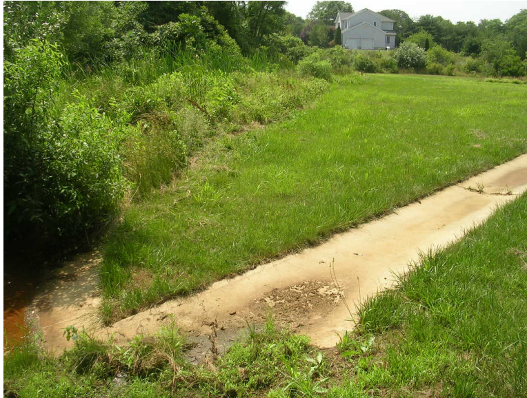
Figure 57. Dry detention basin at station #80, showing turf grass vegetation and concrete low-flow channels, photo taken in summer 2009.
