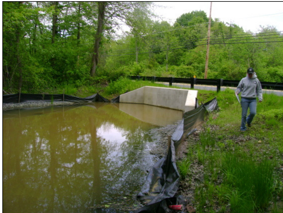
Figure 48. Construction of culvert crossing upgrade at station #63.
