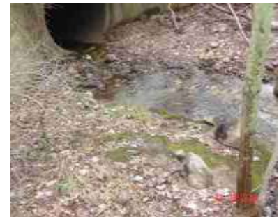
BMP-27 Grouted Rip-Rap Scour Protection
