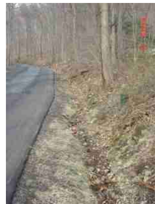
SDO-164 De-vegetated Swale
