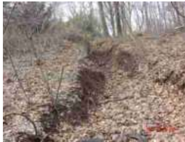
AOC-46: Severe Erosion Downstream of Stormwater Outfall
