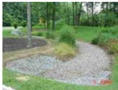
MDB-7: Well Maintained Detention/Infiltration Basin
