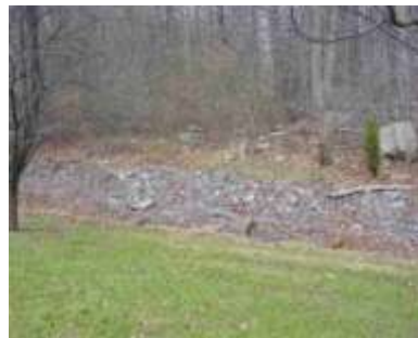
BMP-2 Gabion Stabilized Stream
