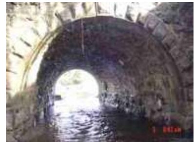
CUL-45 Arched Culvert Under Railroad
