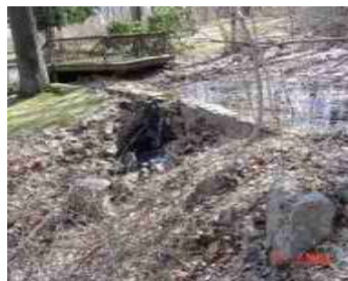
DAM-19 Concrete Dam on Fox Farm Branch
