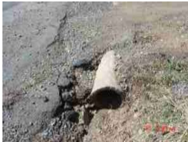
OPG-342 Outfall Pipe with No Conduit Outlet Protection
