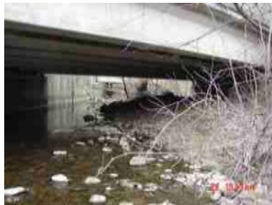
CUL-29 Boxed Culvert and Channel Under Interstate 78
