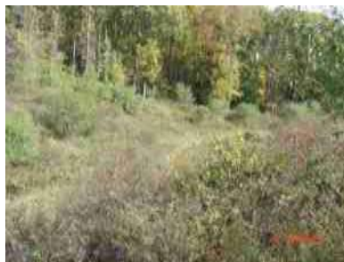
MDB-10: Detention Basin Overgrown with Vegetation
