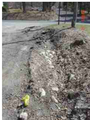
SDO-101 De-vegetated Swale
