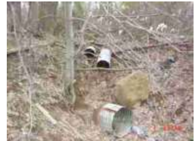
OPG-7 Outfall Pipes With Erosion
