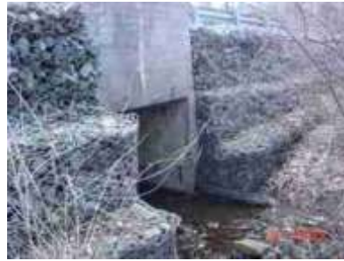
CUL-54 Box Culvert Under Mine Road in Bethlehem Township
