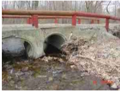
CUL-96 Double Barrel Culvert under Private Road
