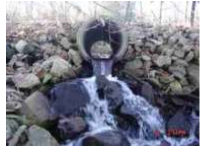
CUL-40 Piped Stream Under Driveway
