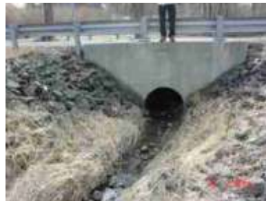
CUL-61 Culvert Under Charlestown Road
