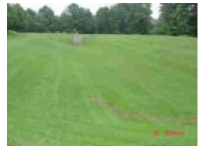
MDB-17: Well Maintained Turf Grass Detention Basin
