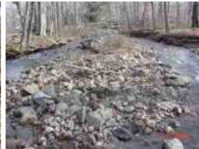
AOC-4: Sediment Deposition in the Stream Channel
