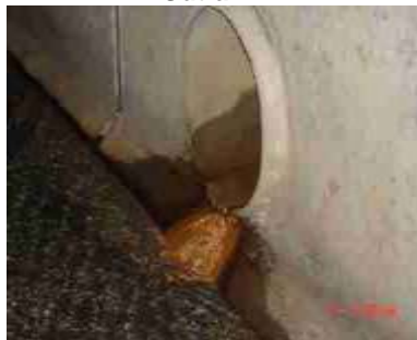
AOC-30 Interstate 78 Drainage with Iron Bacteria
