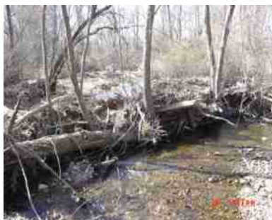
DAM-23 Debris Dam on Charlestown Branch
