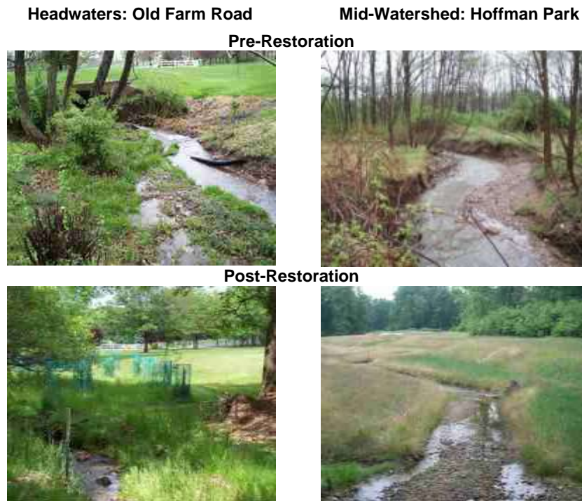
Figure 18. Mechlin Corner Branch Visual Assessment Locations
