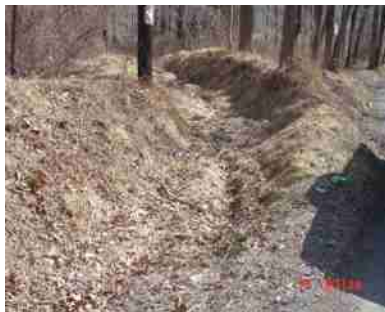
BMP-9 Roadside Drainage Diversion
