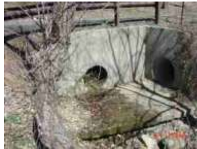
OPG-454 Multiple Outlets with Headwall and Wingwalls
