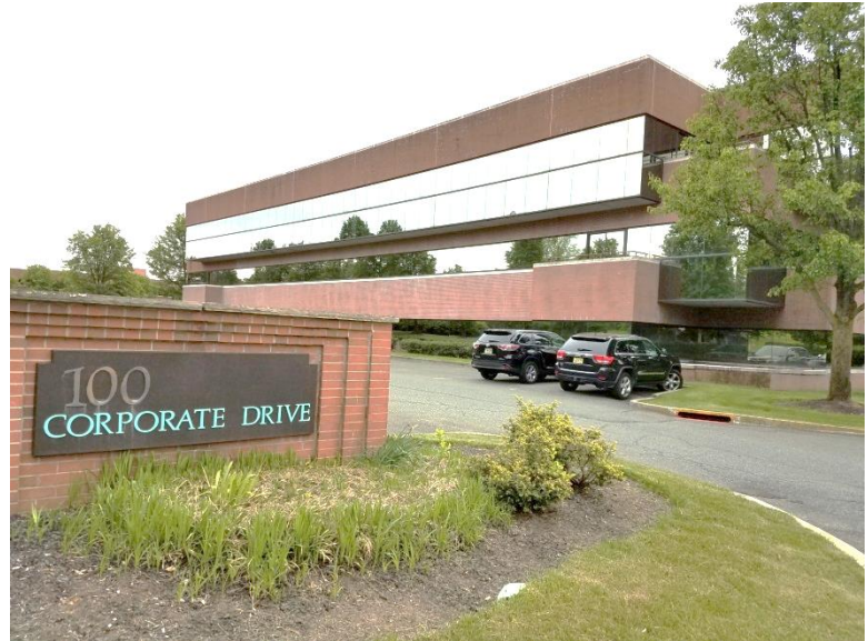
Photo 6: One of the buildings within the office park
