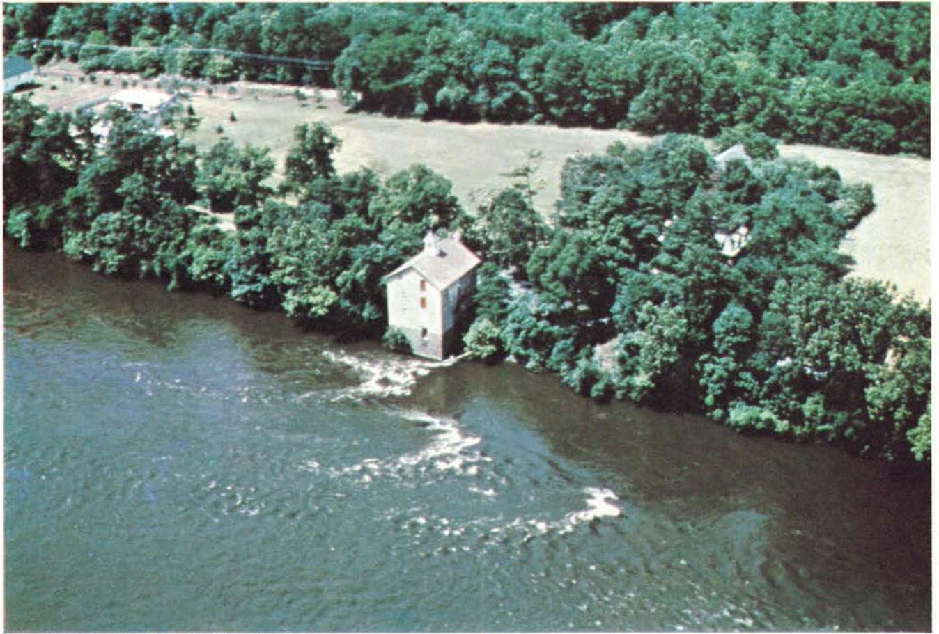
Grist mill at Erwinna, Pa., along the Delaware's main stem.
