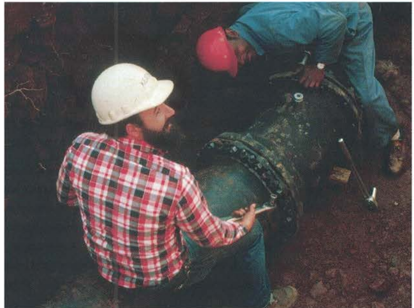
Two workmen repair a leaky water main.
