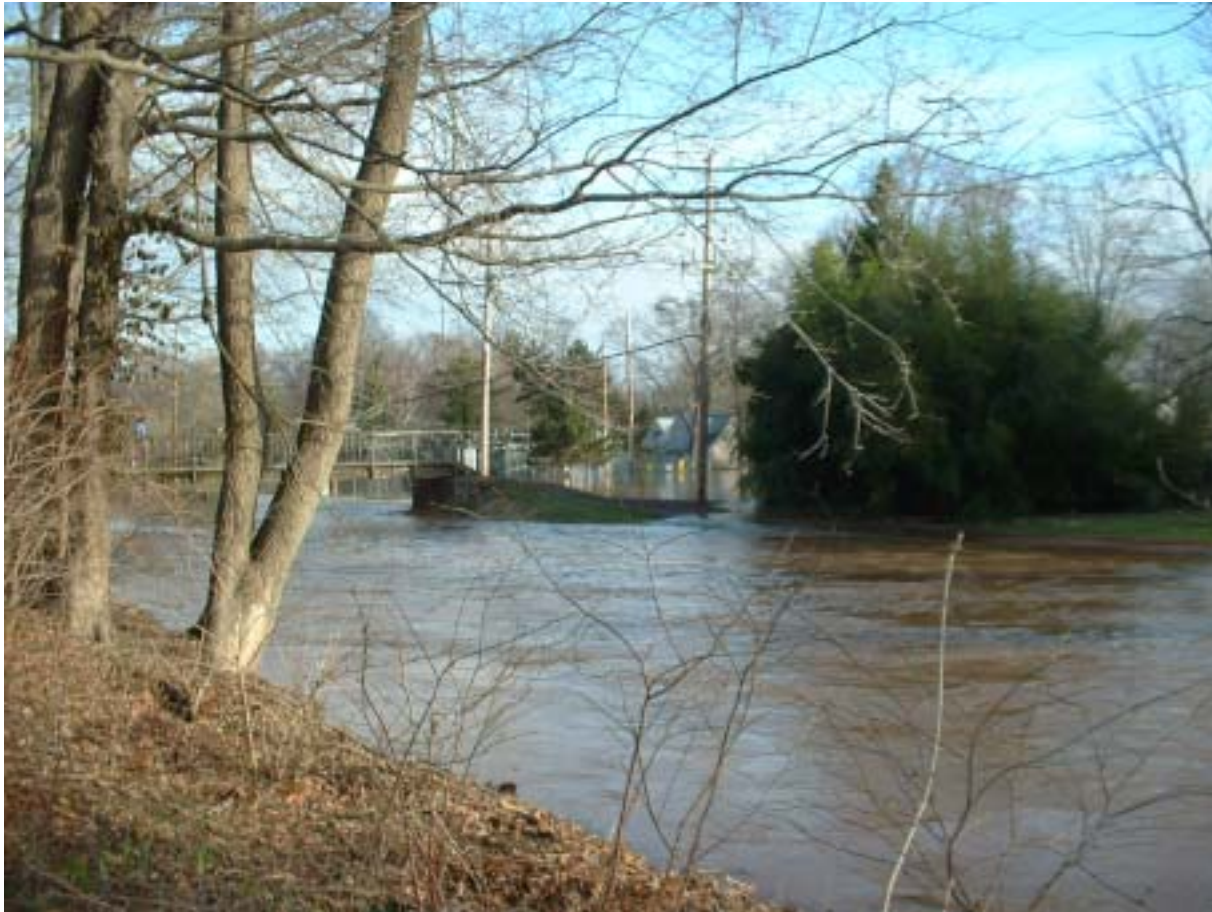
Delaware Canal at Yardley, Pa. – one half mile upstream of Afton Avenue Bridge – 8:30 am, April 4, 2005 Canal bank overtopped by Delaware River. River stage at U.S. Geological Survey (USGS) Trenton gage = 25 ft.
