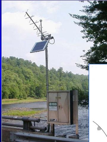
Modern: Pressure Transducer and Electronic Equipment
